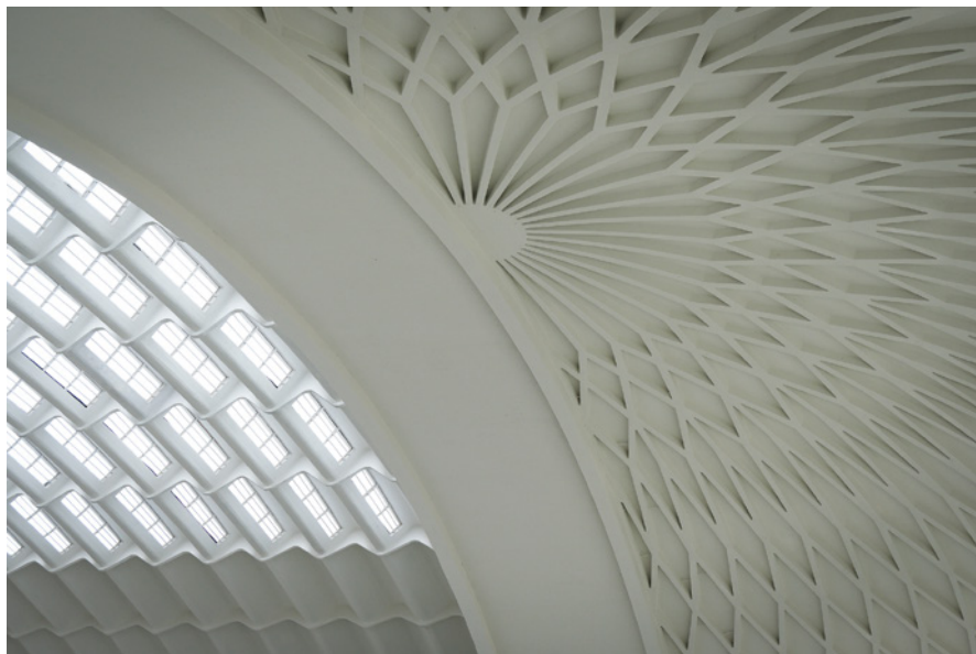
Figure 1 Detail of the vault of the Padiglione Agnelli in Turin during construction works.
