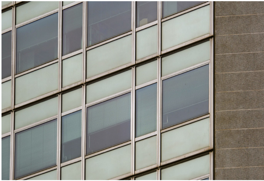
Figure 4 Detail of the curtain wall.
