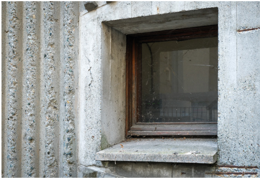
Figure 2 Detail of one of the smaller openings with a pitch-pine window frame.
