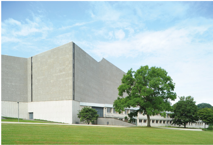
Figure 4 Exterior view of the stage tower and the administration wing, 2016.
