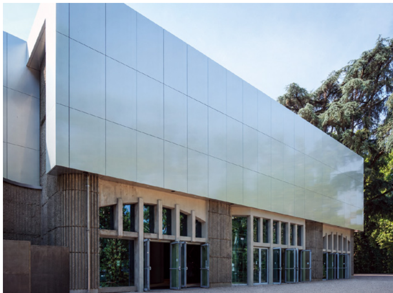
Figure 3 Main elevation during the works.
