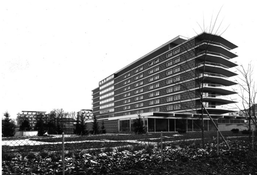
Figure 1 View of the north façade, 1967.
