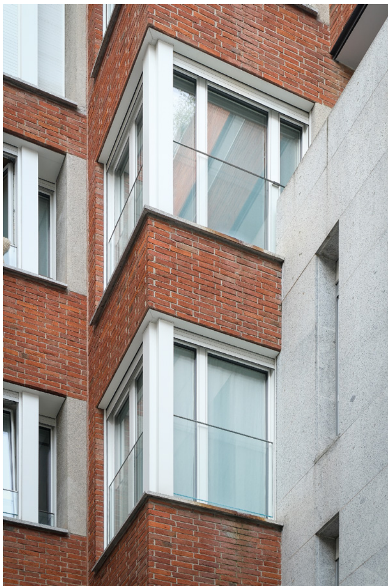
Figure 2 Detail of the main façade of the building on Via Leopardi in Milan.
