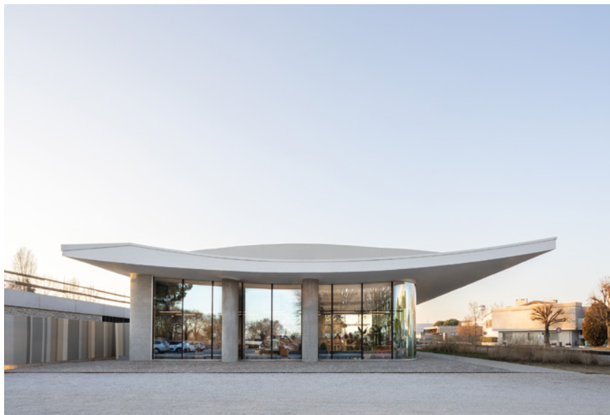
Figure 3 General view after completion of the intervention.
