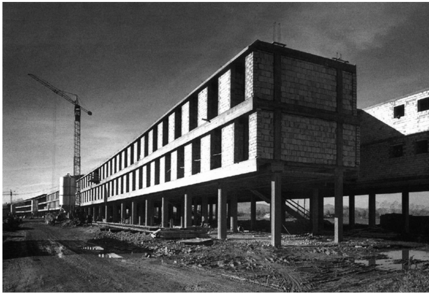
Figure 2 View of the construction site.
