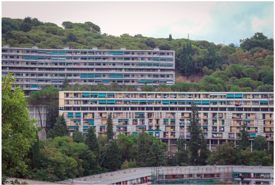
Figure 3 General view upon completion of the intervention.
