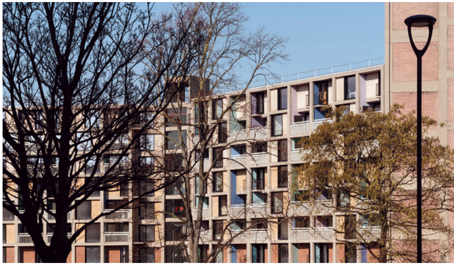
Figure 4 View of the residential façade through the landscaped grounds.
