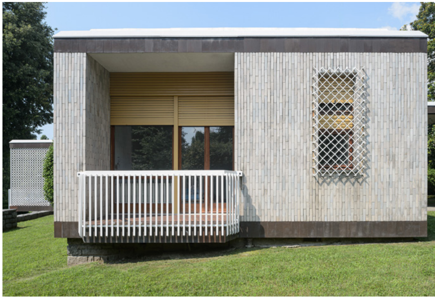
Figure 4 Side façade after restoration.
