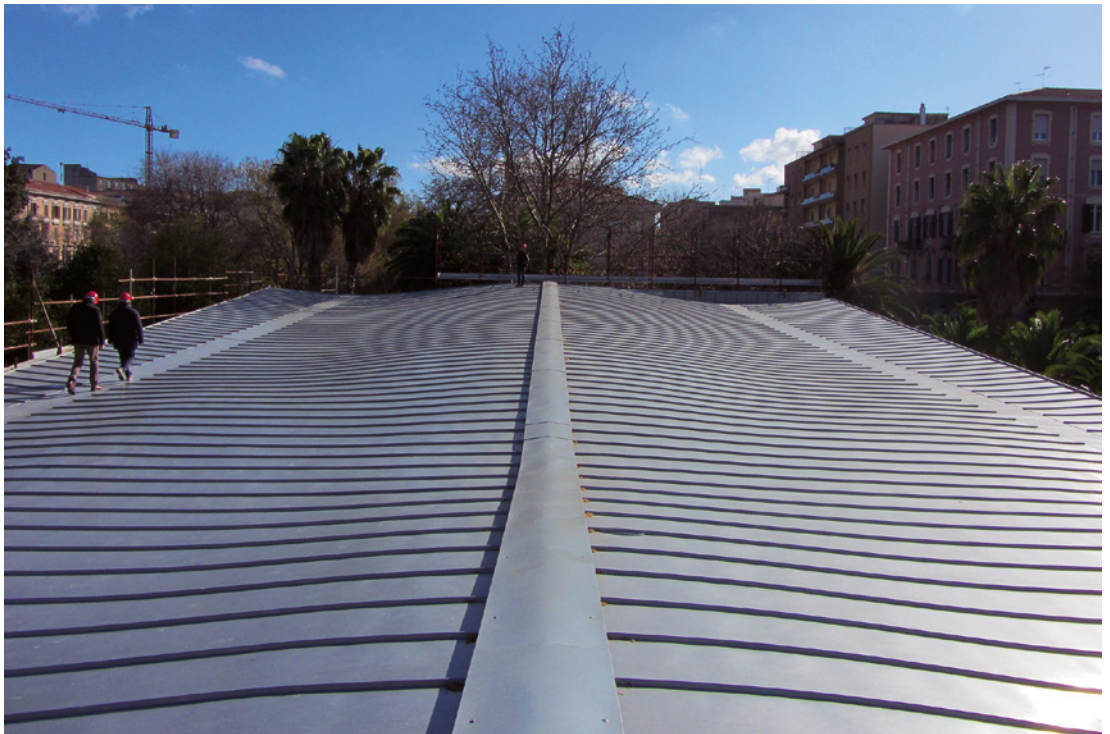
Figure 6 The canopy over the terrace after the intervention.
