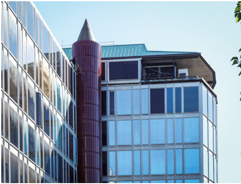
Figure 4 One of the fire-escape stair towers added in 1985, to be removed as part of the intervention.
