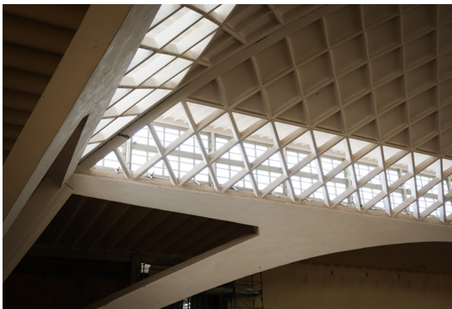
Figure 5 Detail of the junction between the arch and the ribbed roof during construction, 2026.
