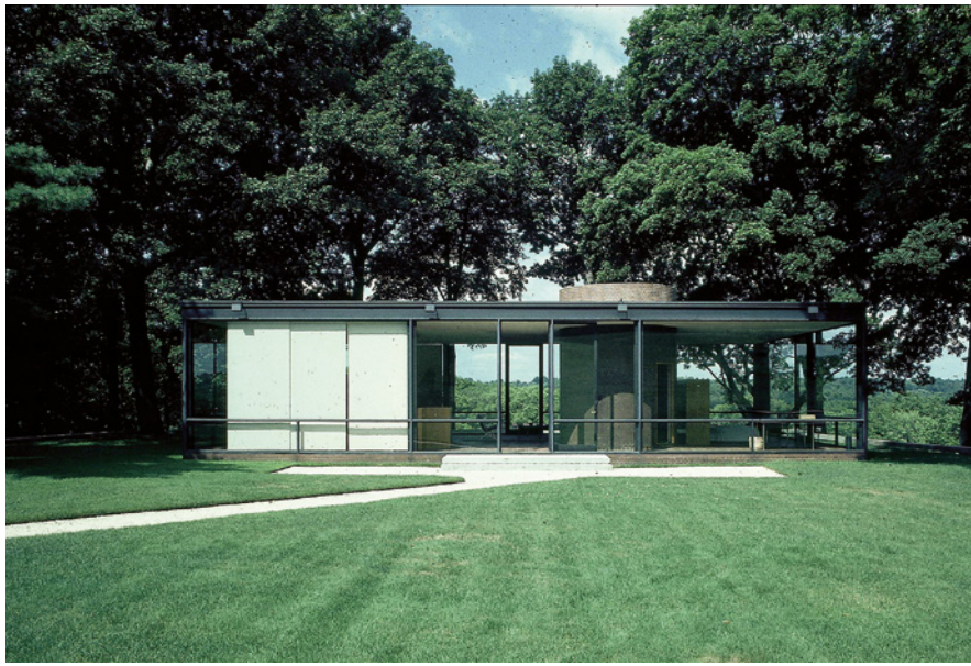
Figure 2 View of the main (east) façade, historical photograph.
