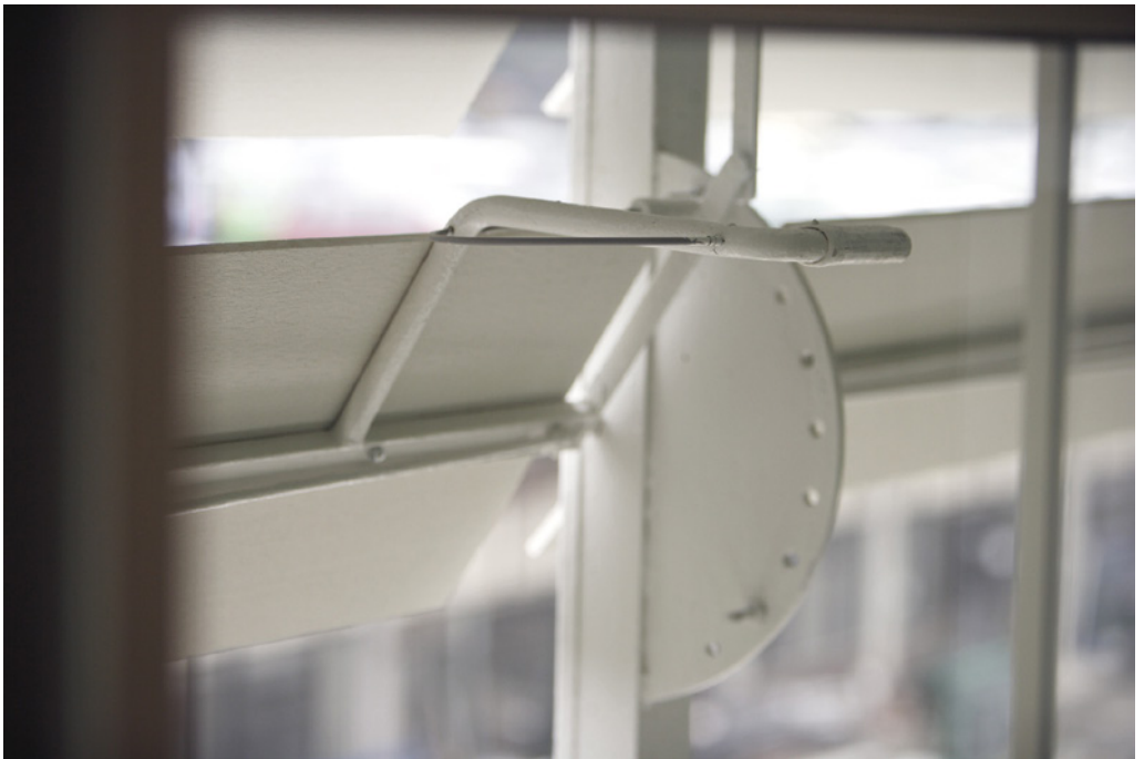
Figure 6 The opening mechanism of the outer façade layer after restoration.
