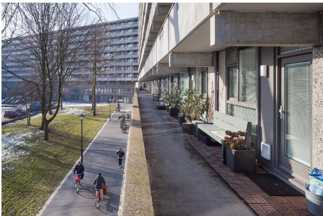
Figure 6 View of the 'reactivated' podium, with new openings and ground-floor spaces.
