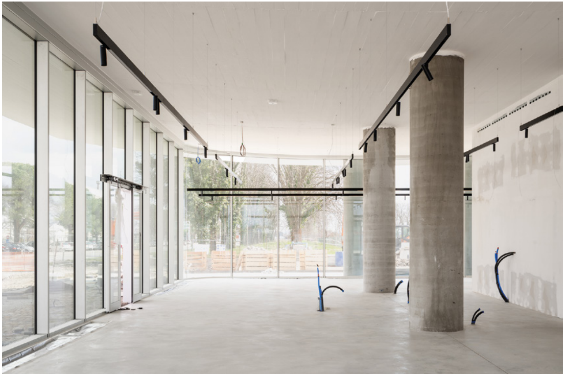
Figure 6 View of the construction site.
