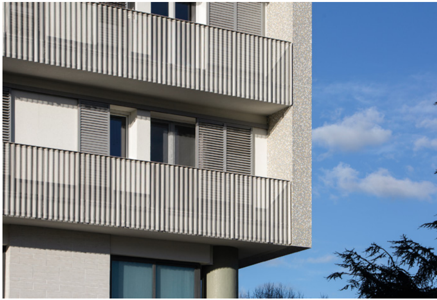
Figure 4 Detail of the loggia with a microperforated sheet-metal balustrade and sliding shutters with adjustable louvres.
