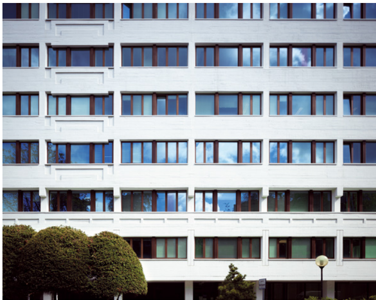
Figure 4 Detailed view of the south façade.
