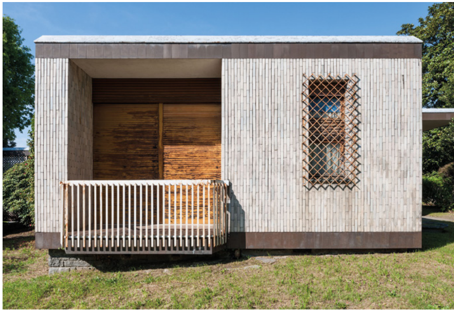
Figure 2 Side façade before restoration.
