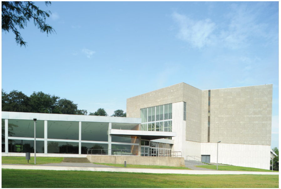
Figure 3 Exterior view of the entrance area, the foyer and the stage tower, 2016.
