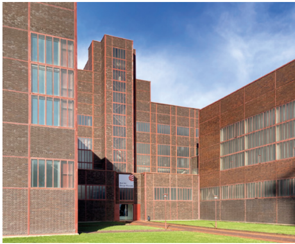
Figure 3 Large steel- and aluminium-framed glazed enclosures characterise many 20th-century buildings from the interwar and post-war periods; photographs from 2014 (top) and 2026 (bottom).
