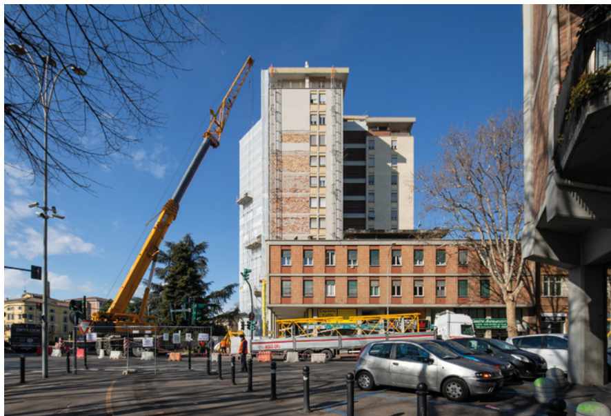
Figure 3 South-east façade with the mosaic cladding removed during the initial stages of intervention.
