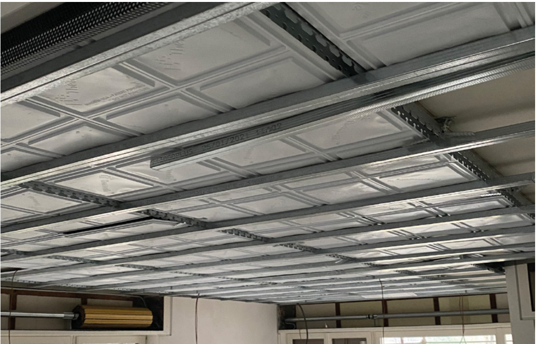
Figure 6 Internal insulation using cork panels.
