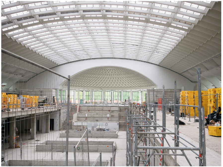
Figure 2 View of the construction site for the new Civic Library within the pavilions of Torino Esposizioni.
