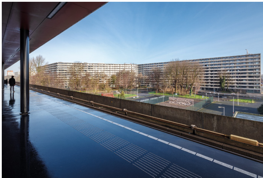
Figure 3 View of the building from the metro.
