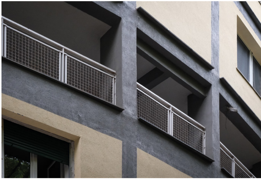
Figure 4 Detailed view of the uphill elevation after the intervention.
