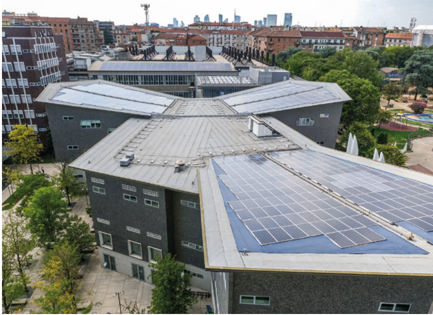
Figure 1 The Trifoglio building at the Politecnico di Milano. The rooftop photovoltaic system was installed on a blue base whose outline echoes the building's plan, visually integrating the installation with the architecture (Photovoltaic System Installation Project for 12 Buildings on the Città Studi Campus, Department of Energy, 2023–2024).
