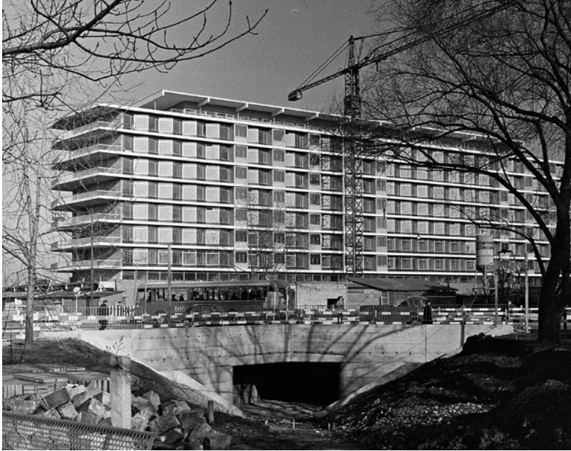
Figure 2 View of the south façade during construction, 1966.
