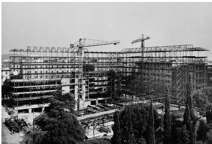
Figure 1 The building's steel structure under construction.
