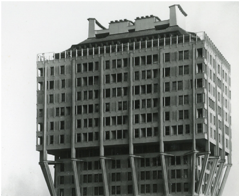
Figure 2 The residential block on floors 19–26, nearing completion.
