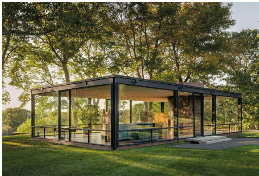
Figure 3 Exterior view of the Glass House from the south-east.
