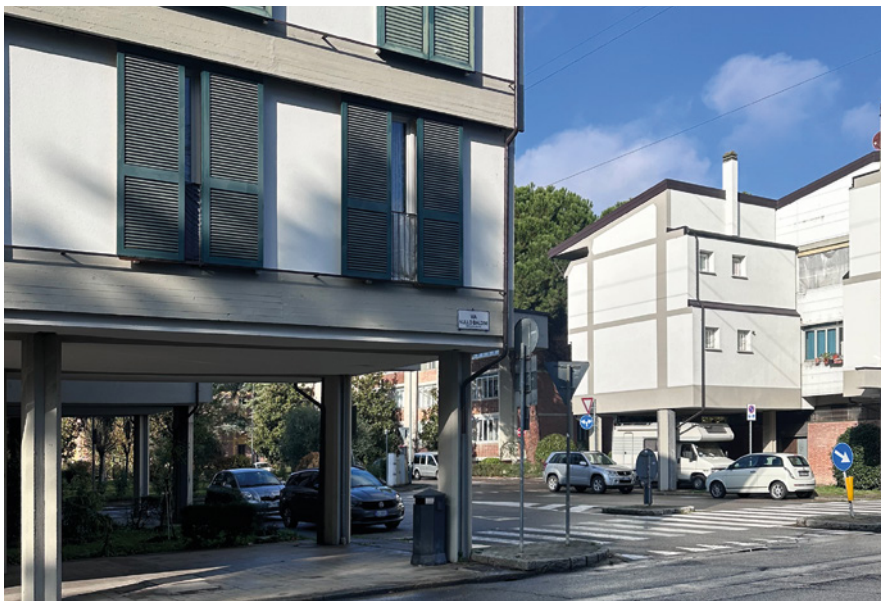
Figure 5 Detailed view after the intervention.
