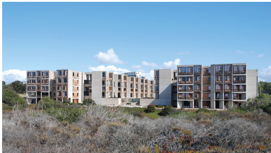
Figure 3 View of the west-facing elevations before work began, 2013.
