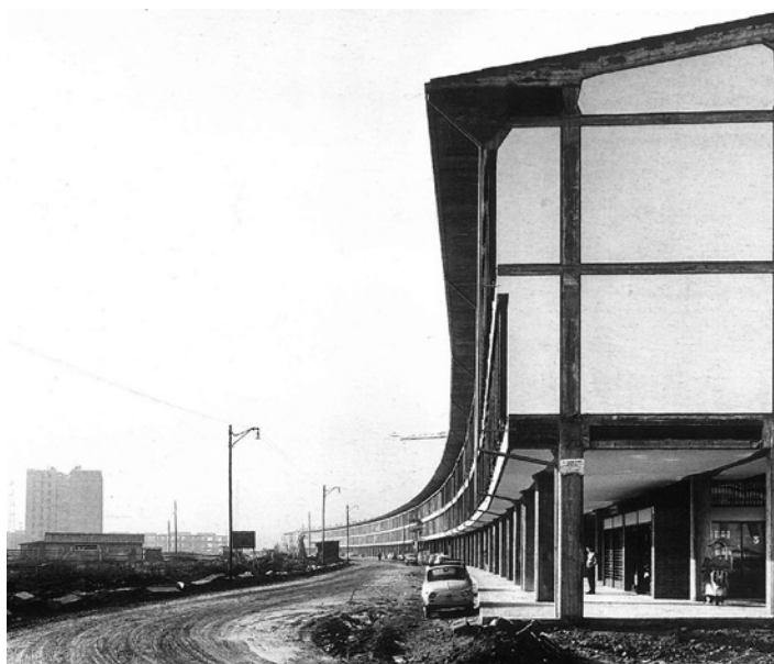
Figure 1 General view of Il Treno, in the still-under-construction Barca neighbourhood.
