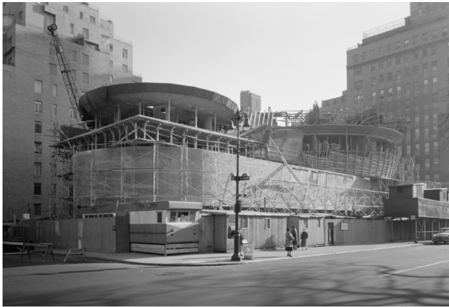
Figure 2 Exterior view of the museum during construction, 1957.
