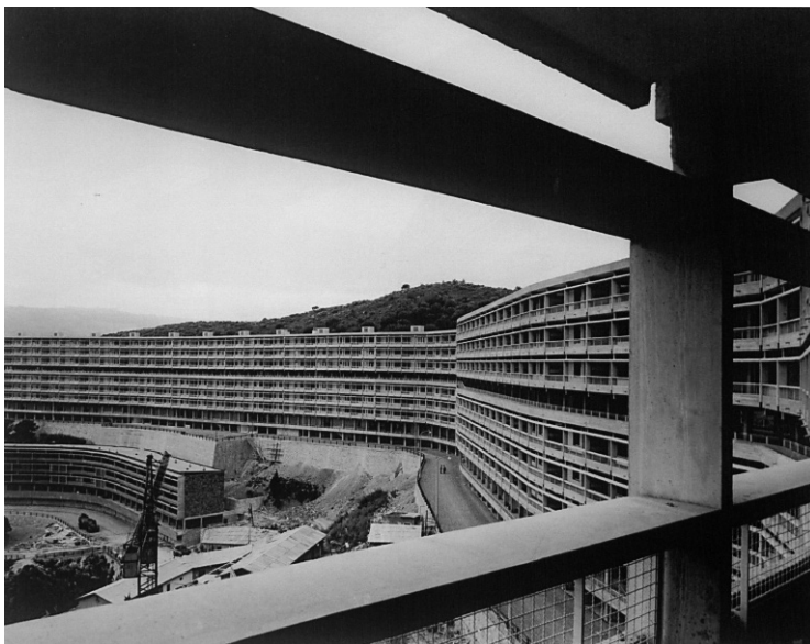
Figure 2 View from the loggia of Building A, looking west.
