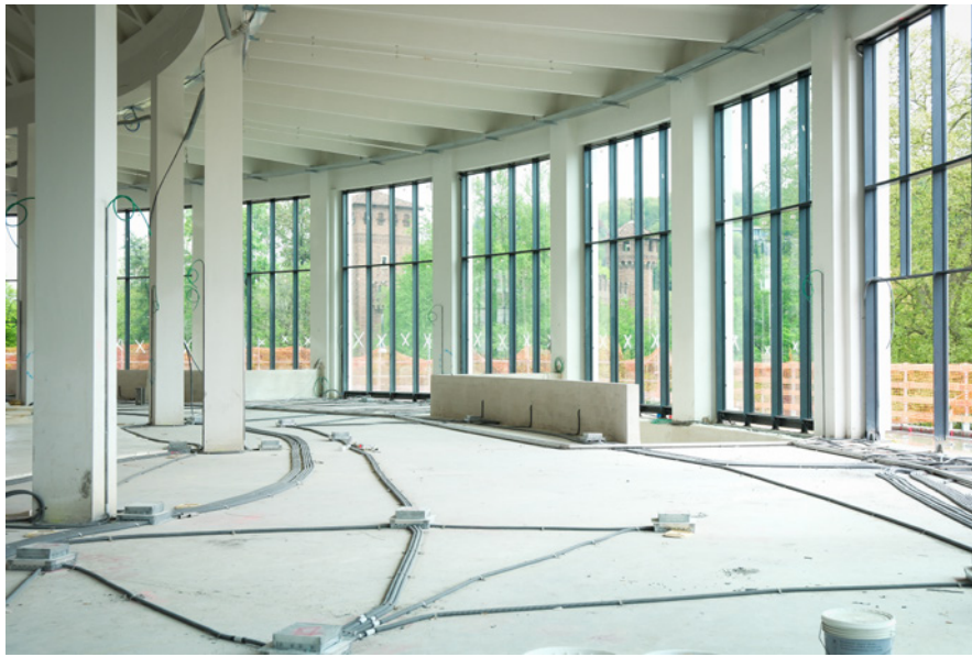
Figure 1 Replacement of the windows in the apse of the Padiglione Agnelli in Turin.
