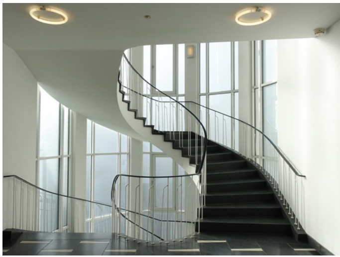
Figure 4 Restored concrete structure and new aluminium-framed glazed enclosure to a stairwell on the rear façade, 2019.
