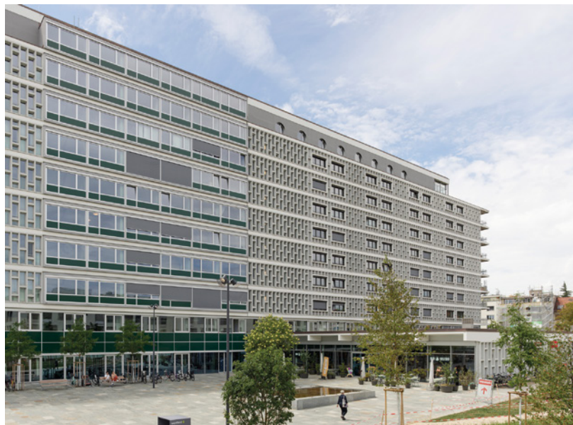
Figure 4 View of the north façade.
