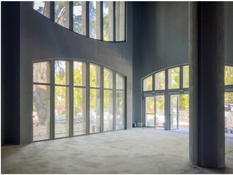
Figure 4 Theatre foyer during the works.
