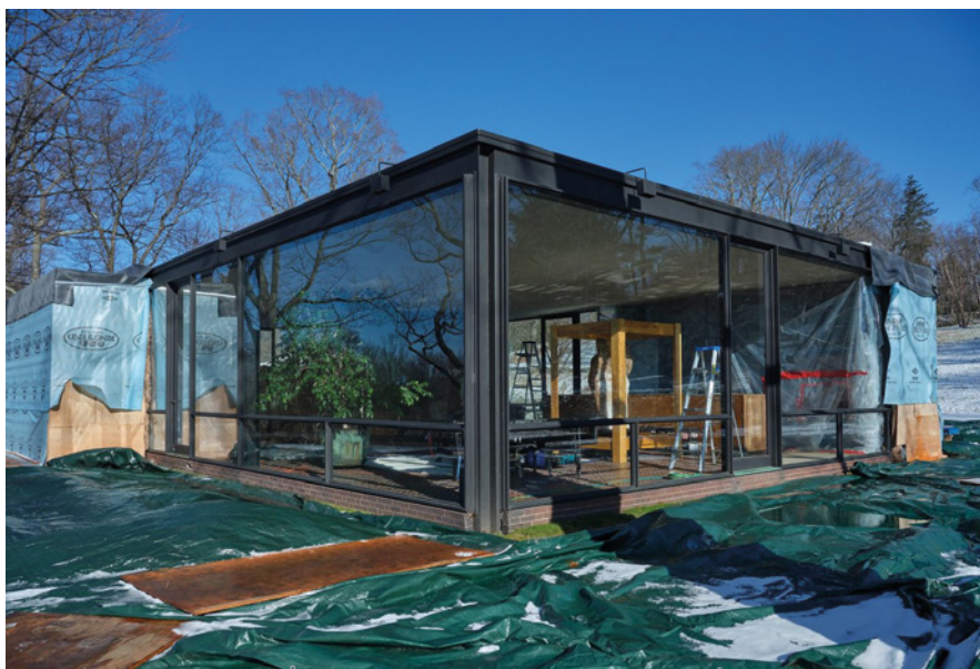
Figure 5 Installation of external protective measures over the cracked glazing, 2019.
