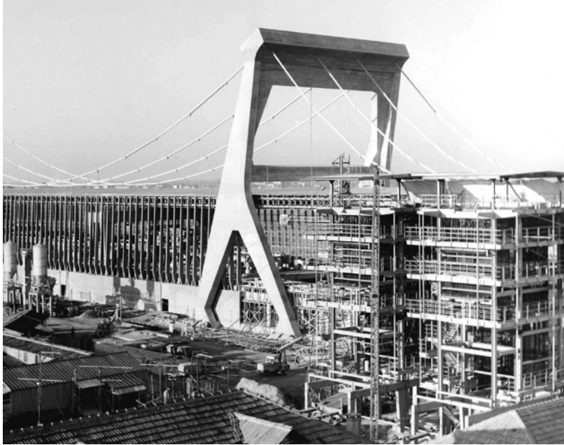
Figure 2 South façade during the installation of the vertical supports and the gas-turbine structure.
