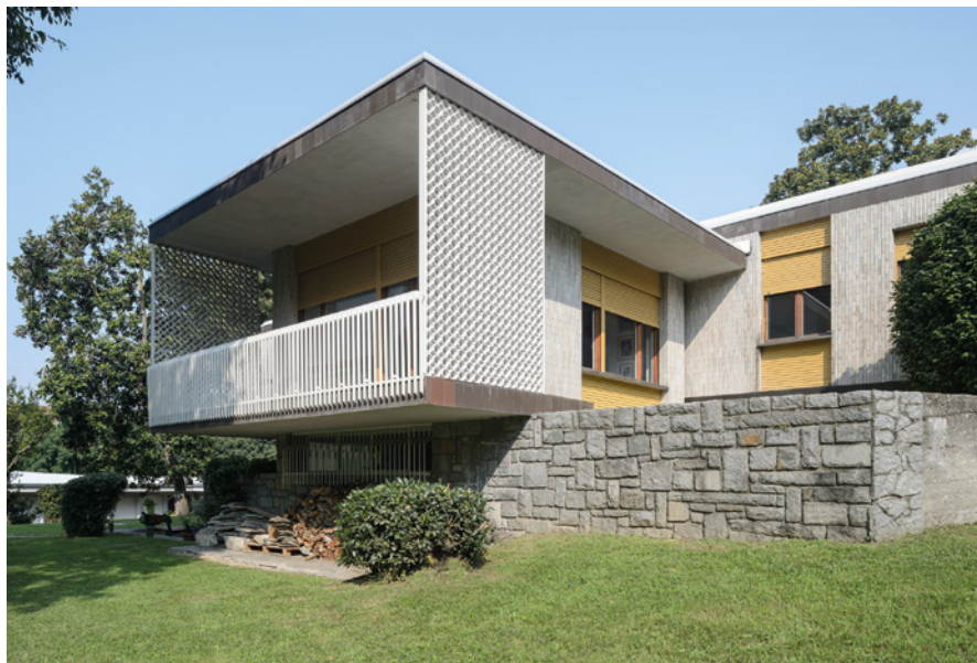
Figure 3 Villa Rossi after completion of the restoration.
