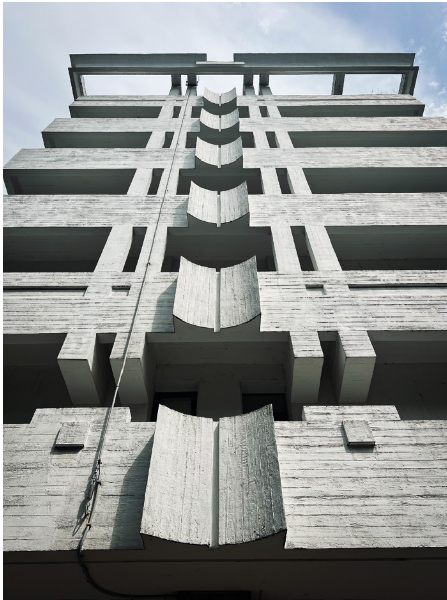
Figure 1 Former headquarters of the Emilia-Romagna Regional Government in Bologna, side elevation.
