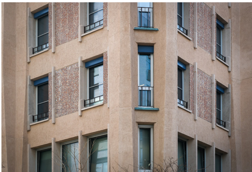
Figure 5 Corner of the tower at the office levels.
