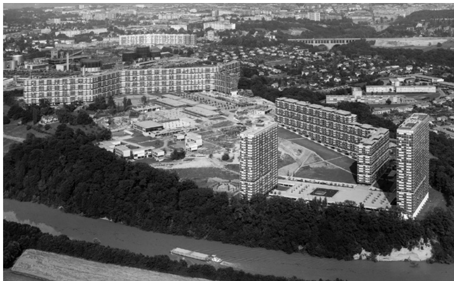
Figure 1 Aerial view of the complex under construction, 1969.
