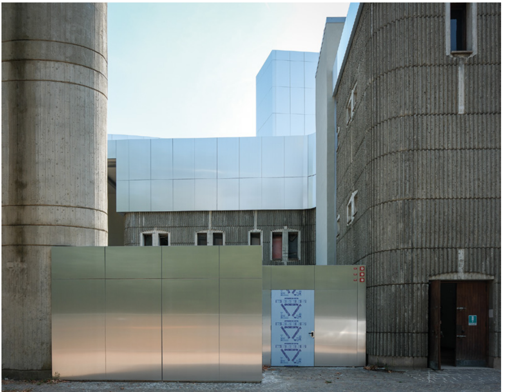
Figure 6 Roof of the theatre auditorium with the new smoke vents.
