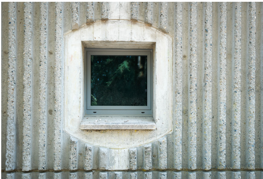
Figure 5 One of the smaller openings with the new window frame.
