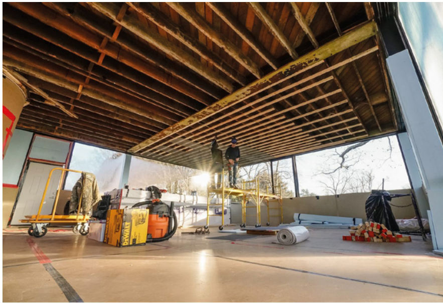
Figure 4 Partial installation of the metal support and suspended-ceiling mesh, 2017.
