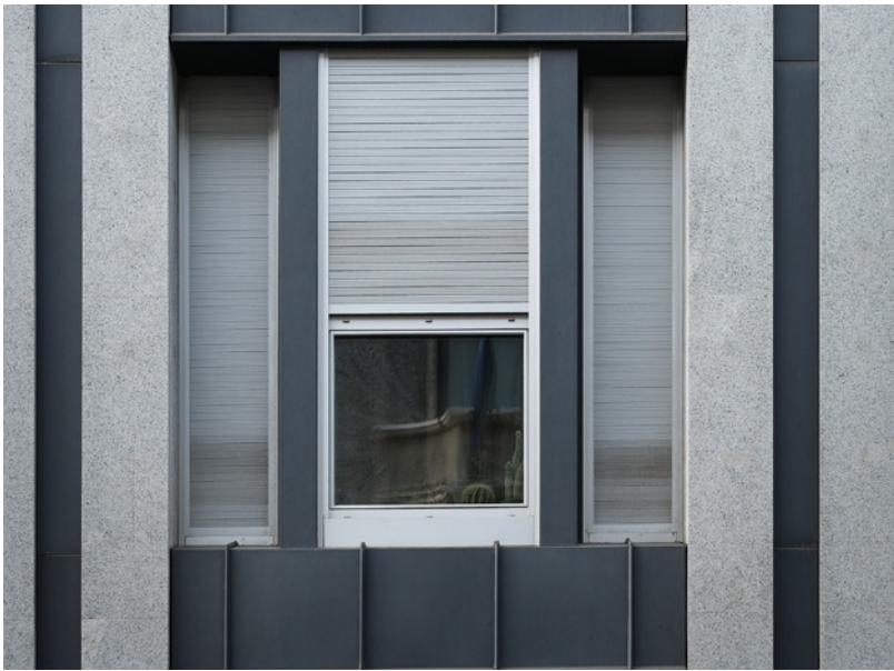
Figure 4 Window frames on the levels originally intended for offices.
