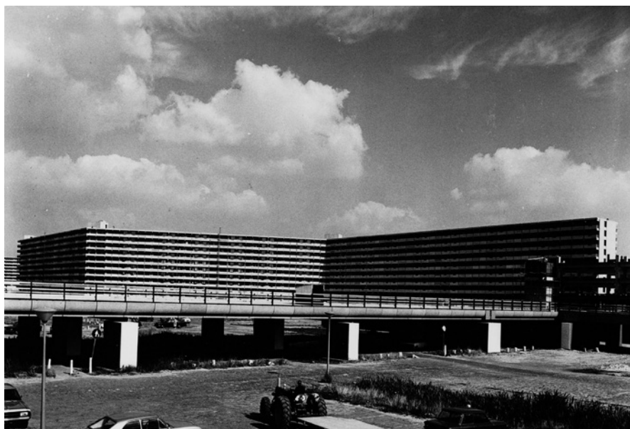
Figure 1 Historical photograph of the building from the south-west.
