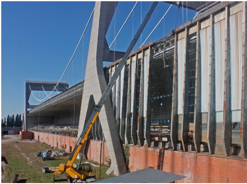
Figure 3 South façade during the dismantling of the vertical supports and panels.
