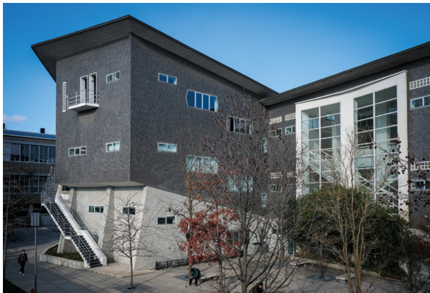
Figure 3 Exterior after the intervention.
