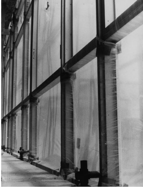
Figure 2 The skyscraper under construction, detail of the façade.
