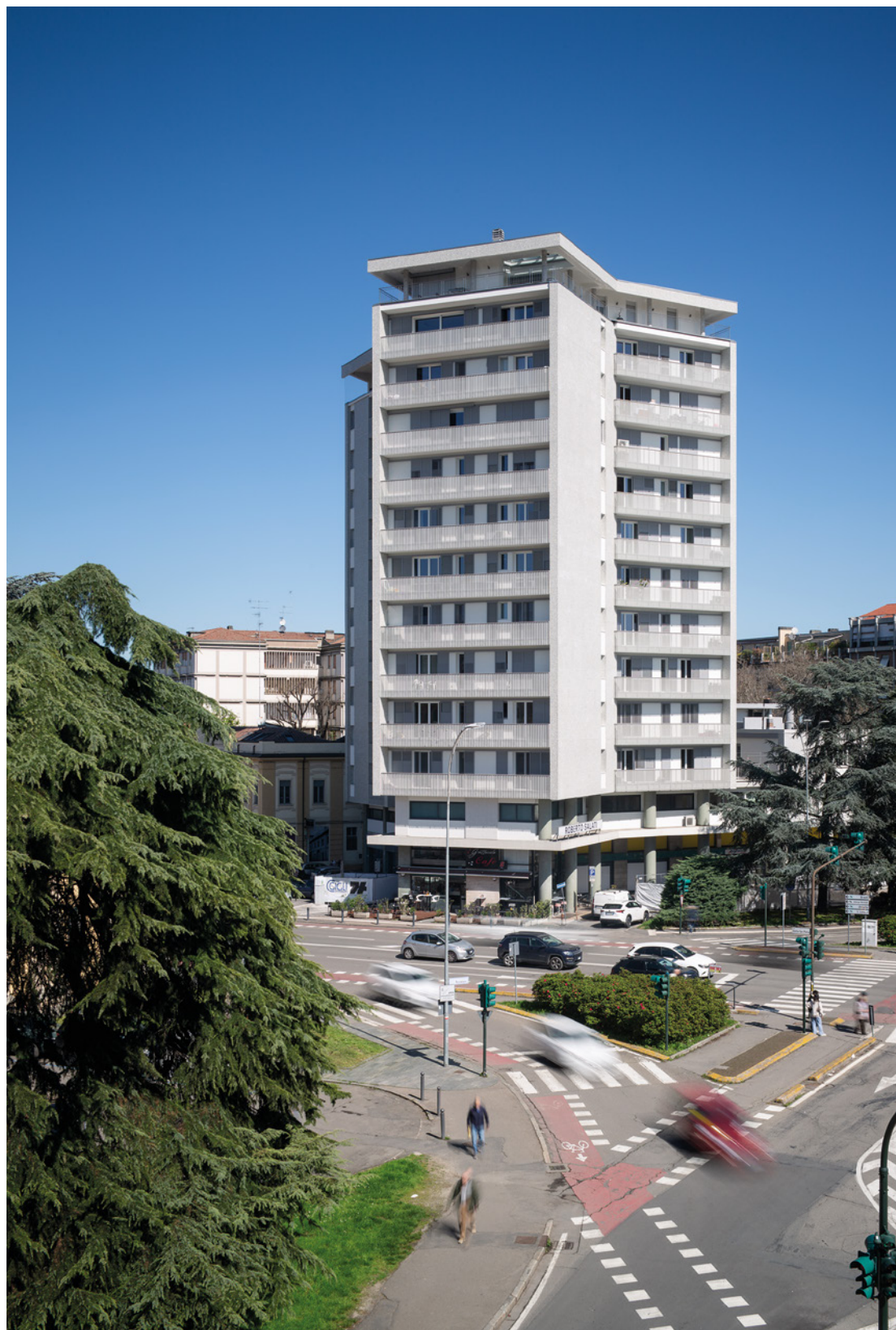
Figure 6 The skyscraper after completion of the intervention.
