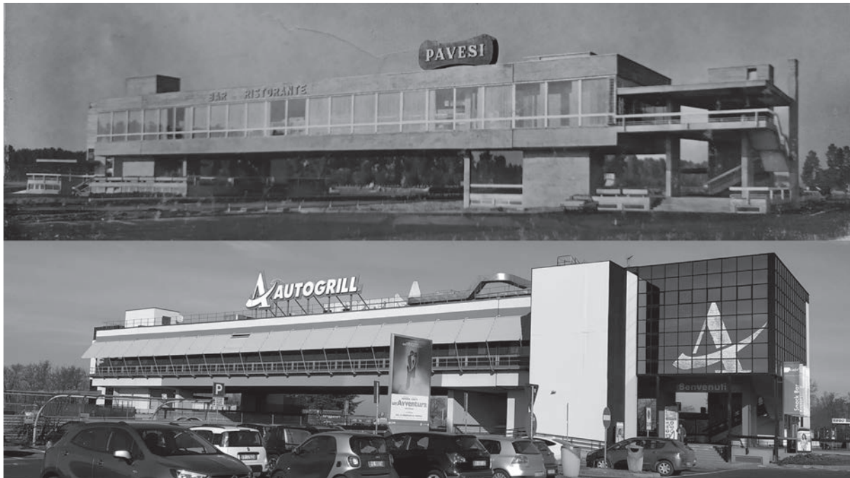
Fig. 3. Autogrill by Carlo Casati in Dorno, Italy, in the 1960s (above) and in 2020 (below). © Carlo Casati archive collection, Politecnico di Milano, Campus Life Area, Library services and archives, Milan; V. Peron, 2020.
