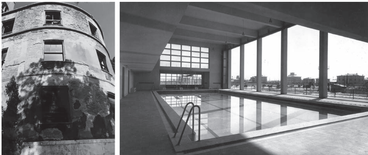
Fig. 2. Cesare Valle, Casa del Balilla, Forlì, Italy. From the left: the co-existence of a reinforced concrete frame with brick masonry; the glazed wall composed of hot rolled steel window profiles and double glazing. © SABAP-RA (Soprintendenza Archeologia, Belle Arti e Paesaggio per le province di Ravenna, Forlì-Cesena e Rimini), Archivio deposito, folder 1 "Fo. Forlì"; AV-Roma, Fotografie, box 25, folder CV-FOT/039.
