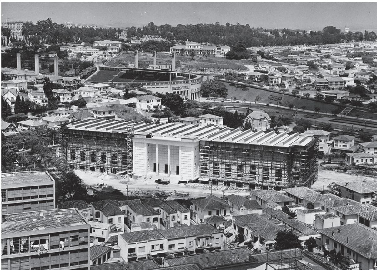
Fig. 3. Auguste Perret, FAAP main building under construction, São Paulo, Brazil, c. 1955. © Arquivo FAAP.
