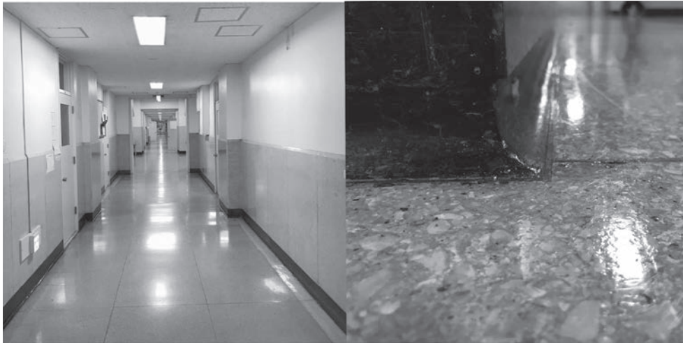
Fig. 3 The corridor of a hall (left). The terrazzo floor and the sanitary base boards (right). © Yu Kishi.
