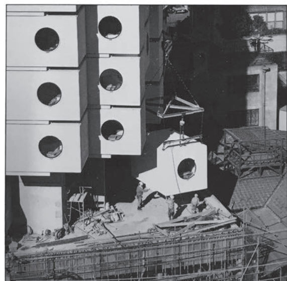
Fig. 1. Attachment of Capsules. © Shinkenchiku-sha.
