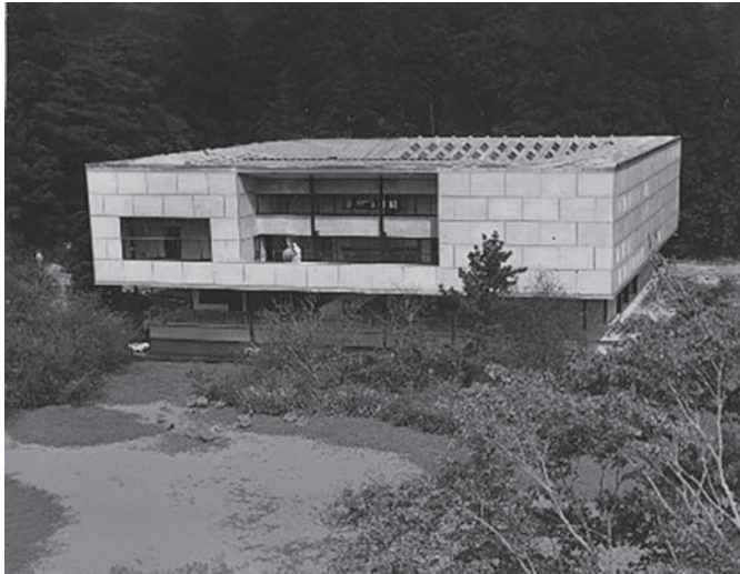
Fig. 3. Museum of Modern Art, Kamakura, pilotis and the drywall materials divided by horse joints were already considered in the project "Ferme Radieuse". 8
