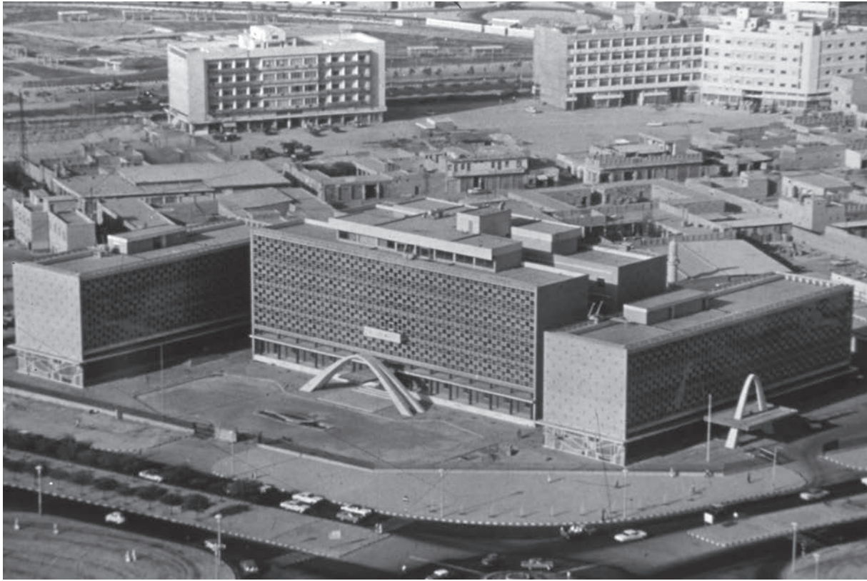
Fig. 3. The Municipality Building in Kuwait designed by Sami Abdul Baki. © Arab Center for Architecture.
