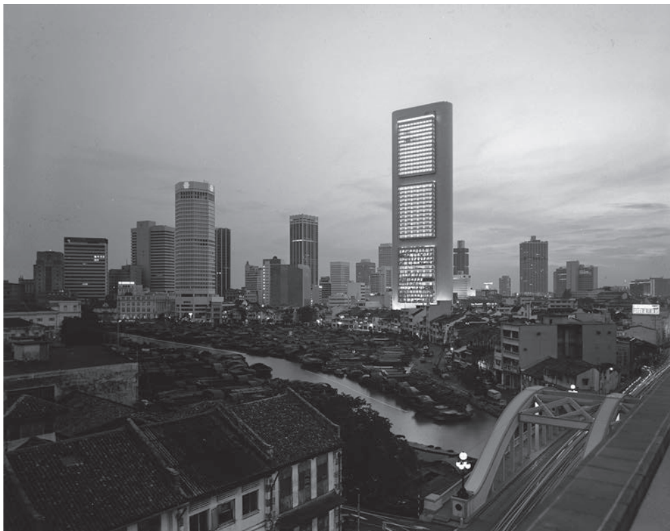
Fig. 2. Urban renewal in progress: newly completed tall buildings midst low-rise colonial vernacular buildings. © Kouo Shang-Wei Collection, National Library Board, Singapore.
