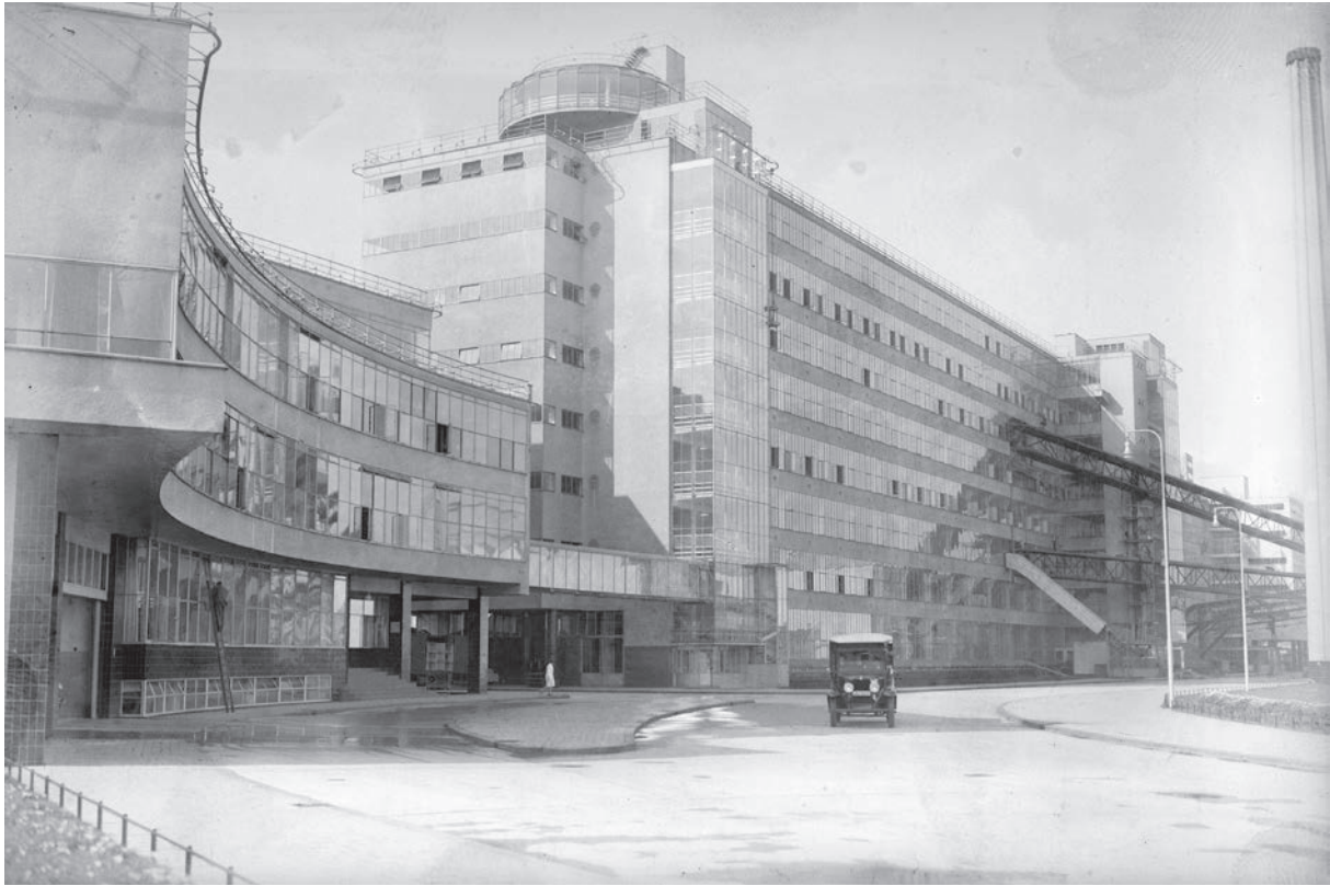
Fig. 1. Jan Brinkman and Leen van der Vlugt, Van Nelle Factory, Rotterdam, The Netherlands, 1927–1930. © Collection Netherlands Heritage Agency, Amersfoort.
