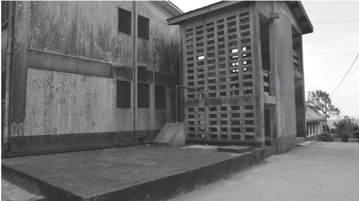
Fig. 1. Dormitory Block, Amedzofe Training College designed by Jane Drew and Maxwell Fry, Image source: © Kuukuwa Manful.
