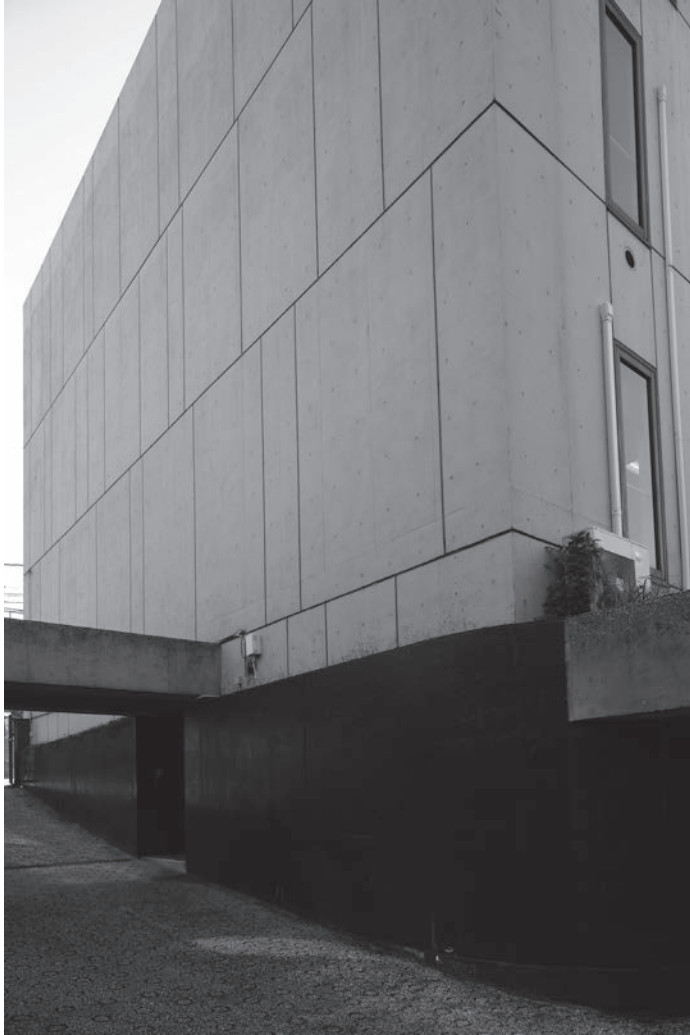
Figs. 1 & 2. Embassy of Brazil, Tokyo. Architect Ruy Ohtake, 1981. © Cristiano Mascaro.
