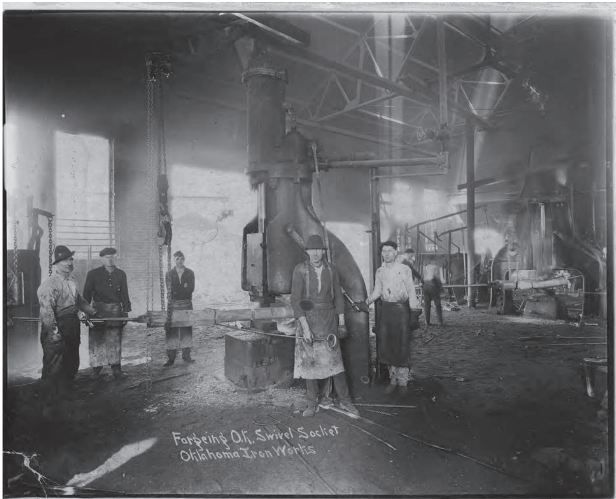
Fig. 1. Forging O. K. Swivel Socket. Oklahoma Iron Works, 1920. © Courtesy of Tulsa Historical Society & Museum, catalogue No. 1975.037.005.
