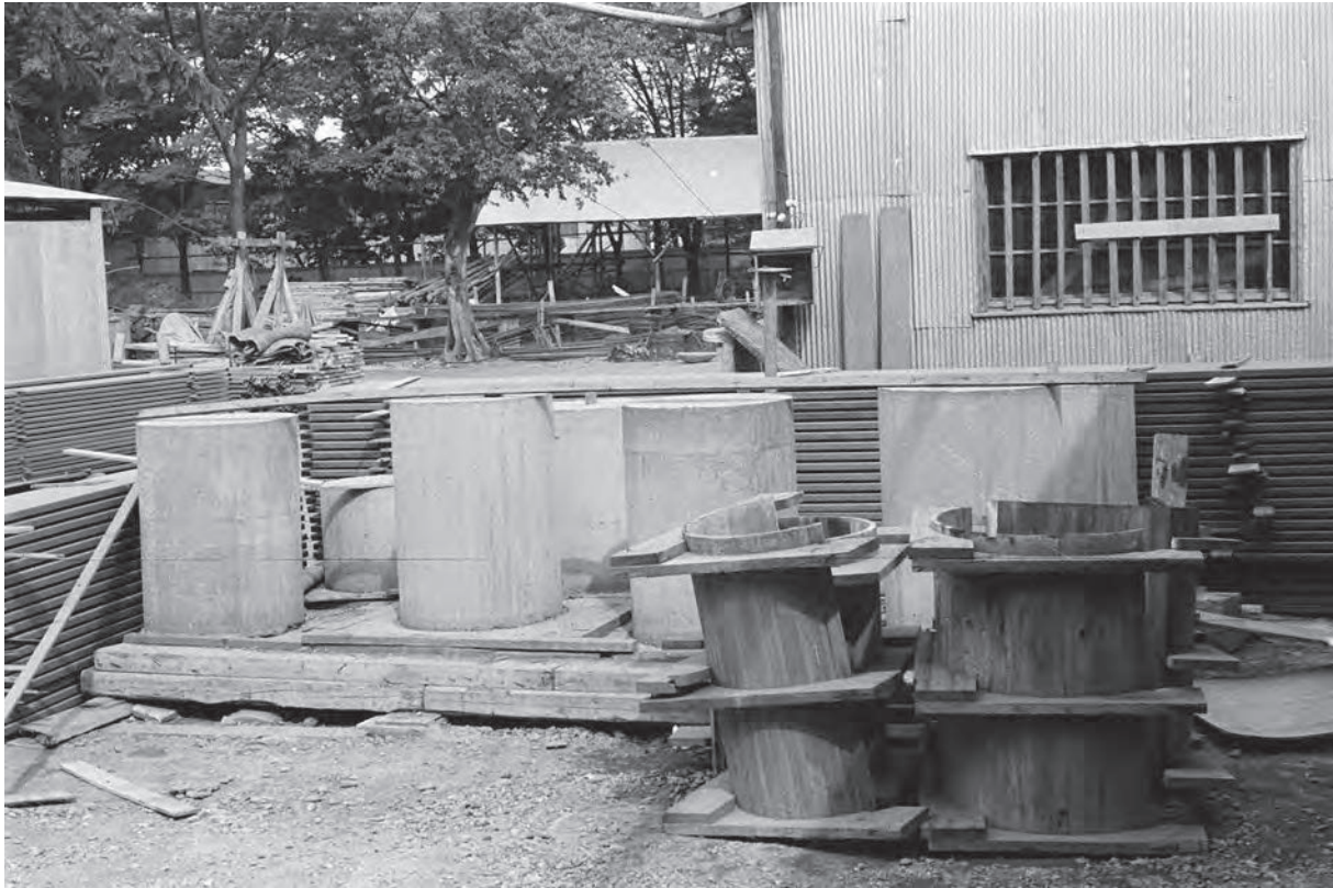
Fig. 2. Le Corbusier, National Museum of Western Art, Tokyo, Japan, 1959, test construction for round columns. © Shimizu Corporation, 1958.
