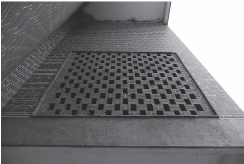
Fig. 4. Po-teh HAN, Municipal Cultural Centre, Changhua, Taiwan, 1983: brick-laying patterns showing the Min-nan style. © Nan-Wei Wu, 2012.
