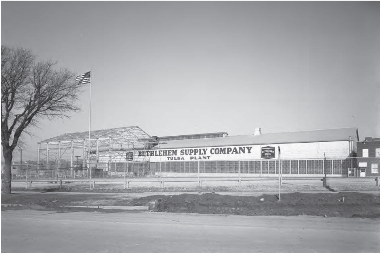
Fig. 2. Exterior of the Bethlehem Steel facility, 1954. © Courtesy of Tulsa Historical Society & Museum.
