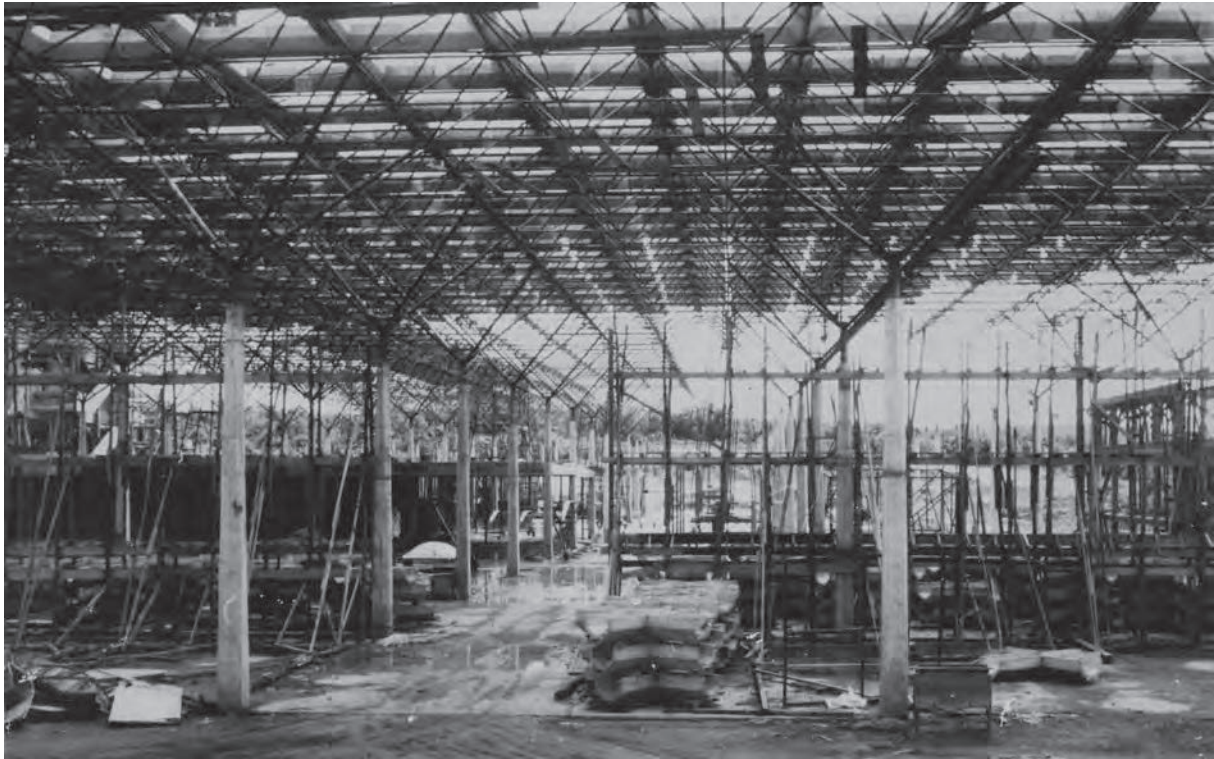
Fig. 2. Amorn Srivongse, Faculty of Engineering, PSU, Songkla, Thailand, 1967–71, by far the most massive space frame under construction. © Amorn Srivongse, c.1969.
