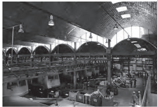
Fig. 3. Dieste y Montañez, Metropolitan Maintenance Plants for Metro Rio, Rio de Janeiro, Brazil, 1976–1978. Interior view. © Hugo Segawa, 2018.
