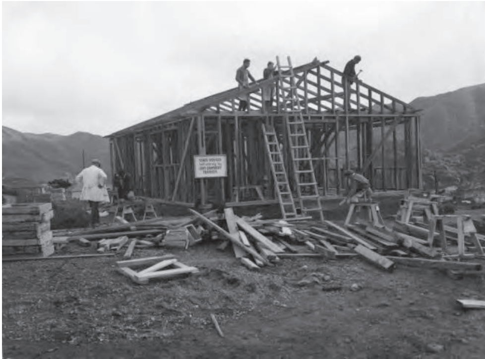
Fig. 1. Building site of a state house showing carpenters at work, Attached to the house is a sign which reads "State houses built entirely by Govt carpentry trainees". © Alexander Turnbull Library, Wellington 1/2-092041-F.
