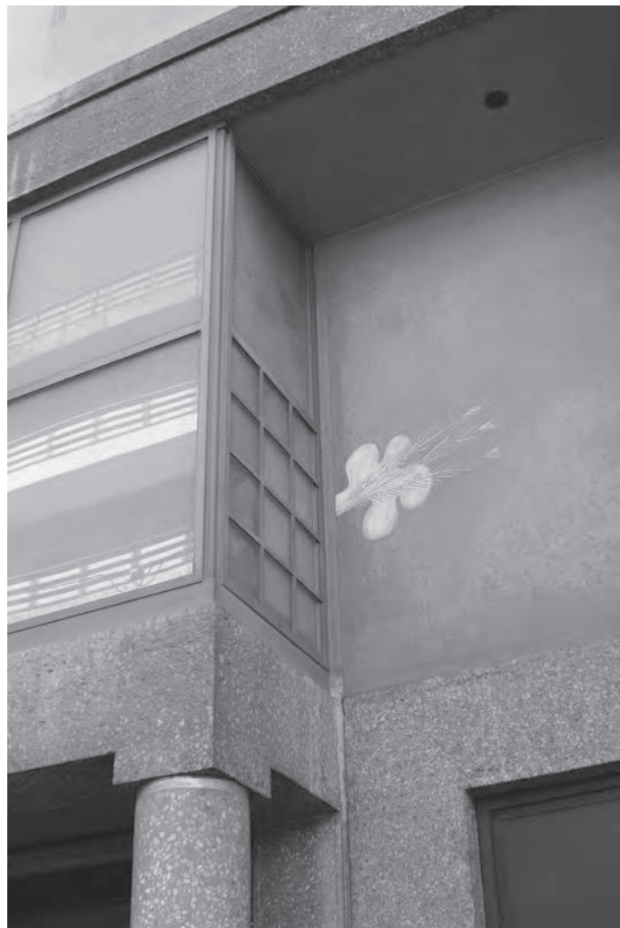
Fig. 3. Kyriakos Krokos, Fassianos Building, Athens, Greece, 1990–1995. © A. Katsakou.
