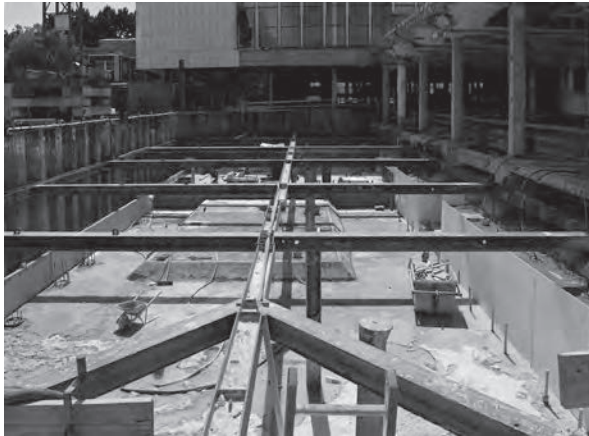
Fig. 3. ARGE Boesch Architekten GmbH / Diener + Diener Architekten / Offermann Architektur & Projekte, reconstruction and renovation Tonhalle/Kongresshaus, Zurich, 2012–2021, temporary horizontal steel supports and vertical steel piles during construction in 2018. © Patrick Fleming, Conzett Bronzini Partner AG.
