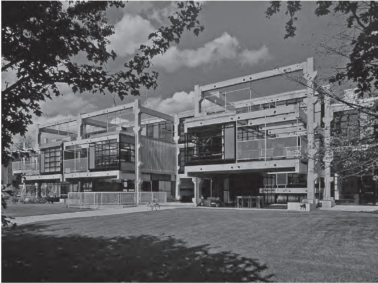
Fig. 1. Genter Strasse 13, Munich, General view of the building on completion of work, S-E front on the street. © Steidle & Partner archive, 1972.
