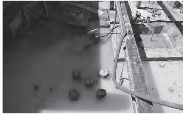
Fig. 4. Haefeli Moser Steiger Architects, Kongresshaus, Zurich, 1937–39, an archival photograph showing the timber piles being driven into the ground in 1937, and a contemporary photograph of five timber piles uncovered during excavation work in 2018. © gta Archives / ETH Zurich, Haefeli Moser Steiger, and Patrick Fleming, Conzett Bronzini Partner AG, respectively.
