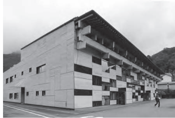
Fig. 1. Kengo Kuma, Yusuhara Town Hall. Main façade. © Ariel Genadt, 2015.
