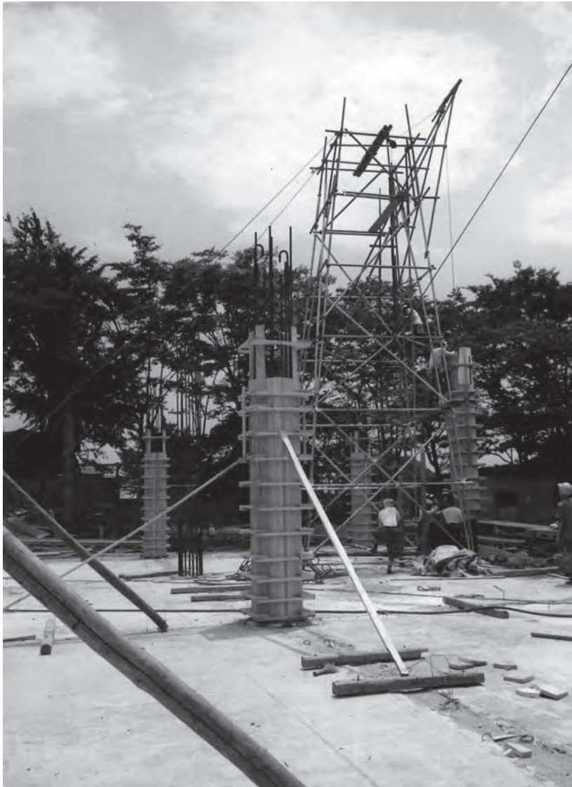
Fig. 3. Le Corbusier, National Museum of Western Art, Tokyo, Japan, under construction of round columns. © Fumio Takano, 1958.
