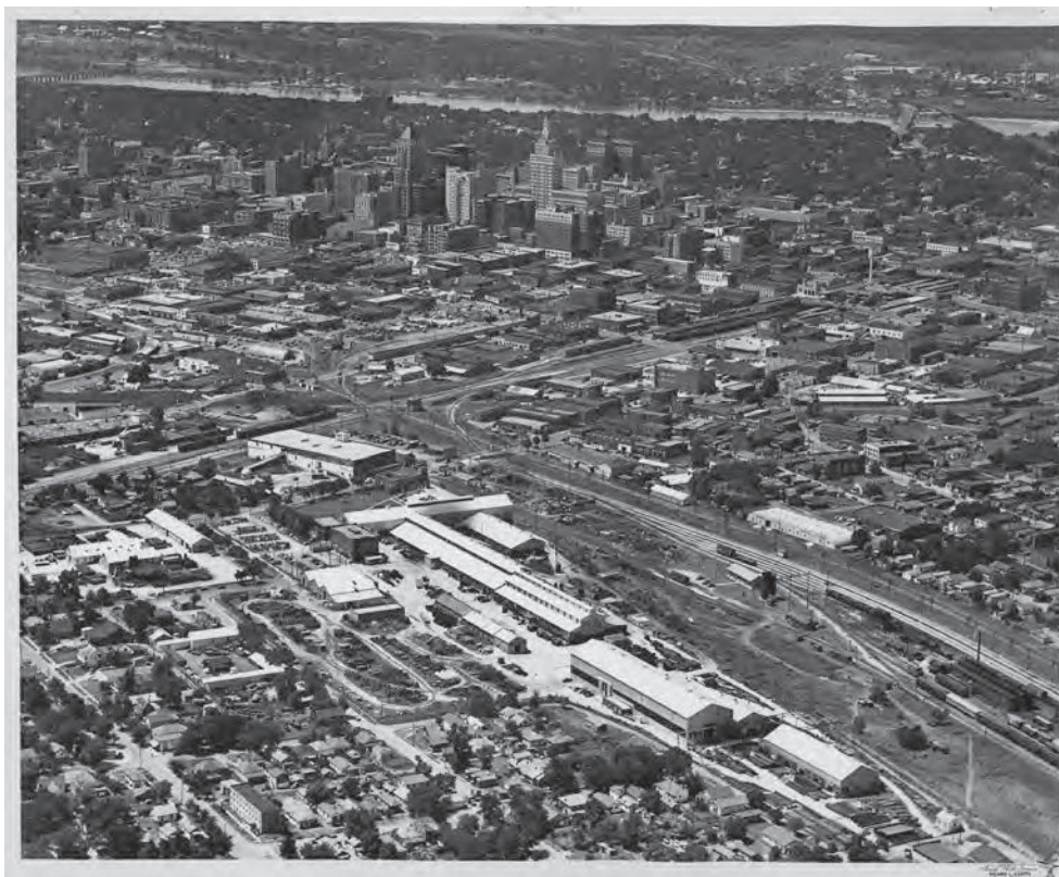
Fig. 3. Aerial view of the Bethlehem Supply Company Tulsa Plant buildings, 1949. © Courtesy of Tulsa Historical Society & Museum, catalogue No. 2006.098.010.
