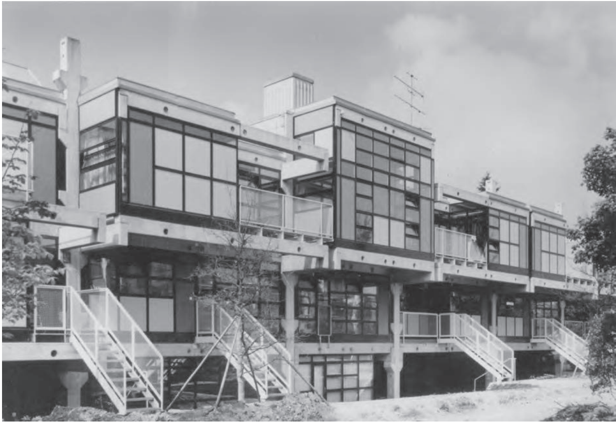
Fig. 3. General view of the whole on completion of work, N-E front on the park. © Steidle & Partner archive, 1972.
