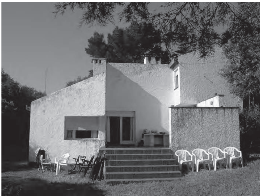
Fig. 3. Albarraque House, 1961, Raul Hestnes Ferreira. Outdoor view of the south courtyard (current state). © João Santa Rita.
