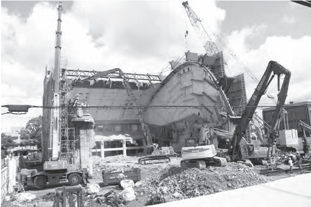
Fig. 1. Demolition of Miyakonojo Civic Hall, October 25, 2019. We posted a daily picture of the Hall on Facebook. ©Yuko Kawagoe.
