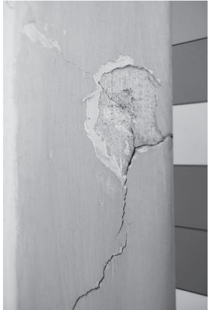
Fig. 3. Damage in the yellow cylindrical wall of the white atelier shows the previous layers_ 2018_ Mariël Polman, RCE.
