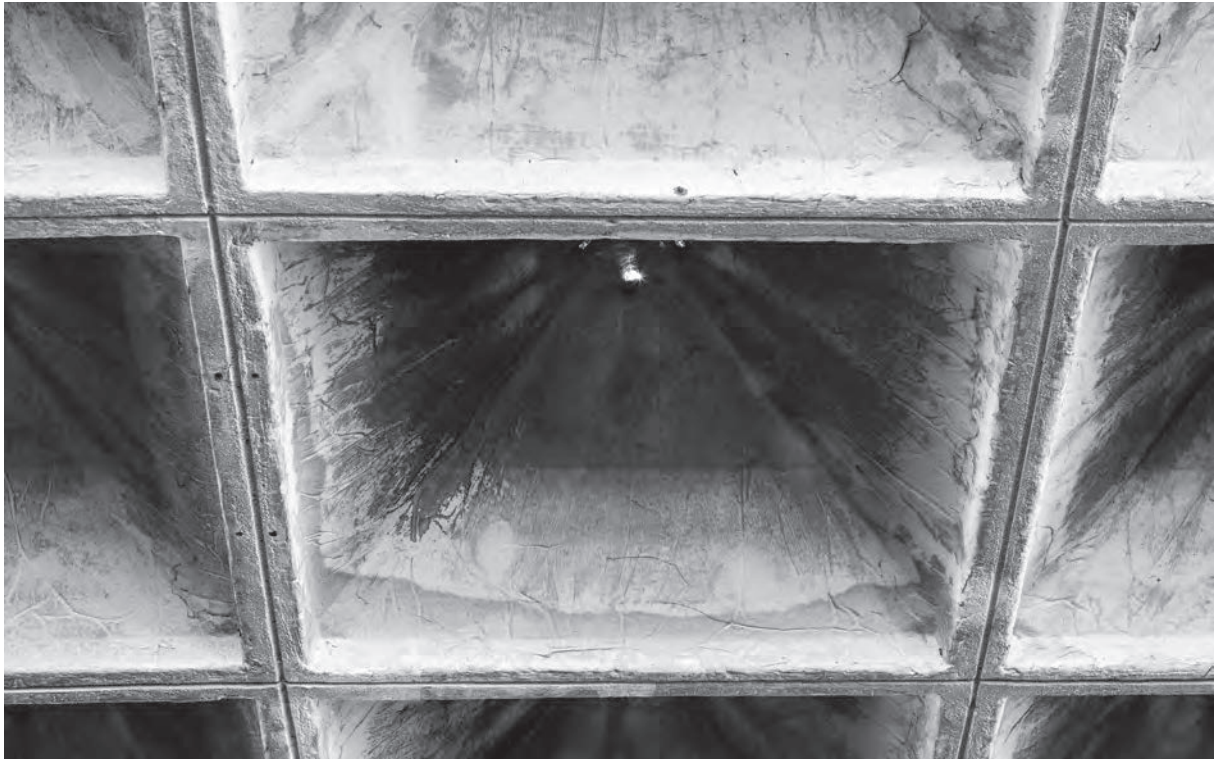
Fig. 4. Amorn Srivongse, Faculty of Engineering, CMU, Chiangmai, Thailand, 1971–73, underside surfaces of precast pyramid roof units left fair-faced. © Sithisak Namkom, 2019.
