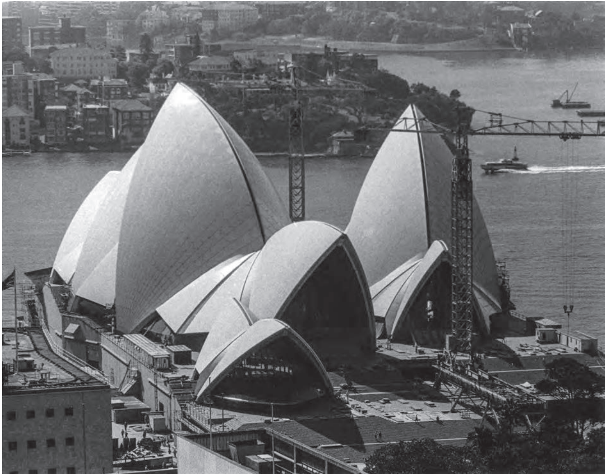
Fig. 2. Sydney Opera House under construction. © Photographer M. A. Lewi, date unknown.
