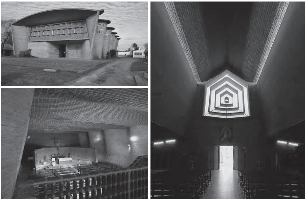
Fig. 1. Church of Christ The Worker, Atlántida, Uruguay, 1960 (left). The Church of Christ the Worker combines two types of reinforced ceramics solutions: the roof in doubly-curved (gaussian) vaults, spanning approximately 16 meters and the undulating walls, seven meters high. The interior space is dominated by the undulations of the ceiling and walls, without, however, losing the sense of order and spatial clarity. Strategically arranged openings bring filtered light to the interior, sometimes colored by the stained-glass windows, sometimes by the onyx membranes in the choir. The altar walls, with different bricklayings, create a special background texture for the image of the crucified Christ. Church of San Pedro, Durazno, Uruguay, 1971 (right). They maintained the idea of a basilica floor plan with three naves, however as a constructive solution, flat slabs of reinforced ceramics were chosen for the walls and roofing. The ceramic slabs, with ingenious folds, articulate side walls and ceiling and, due to the angles, reinforce the perspective of the faithful from the entrance toward the contemplation of the altar. Opposite to it, above the entrance, another expressive element of the church rewards the faithful as they leave the enclosure: a brick rose window delicately supported by thin metal bars, imperceptible due to the contrast between light and shadow. © Hugo Segawa, 2018.
