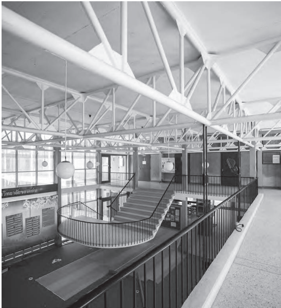
Fig. 1. Amorn Srivongse, Faculty of Engineering, KKU, Khon Kaen, Thailand, 1964–66, suspension structure is lifting the walkway at central hall. © Si-thisak Namkom, 2019.
