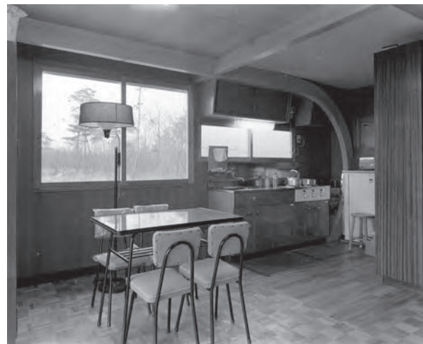
Fig. 2. Gorozo Iizuka, U House, Japan, 1961, a small house with U shape laminated wooden arch. Permitted to publish by Masayuki Miyabayashi.
