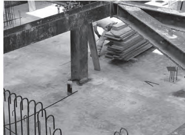
Fig. 3. ARGE Boesch Architekten GmbH / Diener + Diener Architekten / Offermann Architektur & Projekte, reconstruction and renovation Tonhalle/Kongresshaus, Zurich, 2012–2021, temporary horizontal steel supports and vertical steel piles during construction in 2018. © Patrick Fleming, Conzett Bronzini Partner AG.
