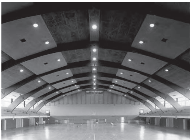
Fig. 1. Gorozo Iizuka, Shibata City Gymnasium, Shibata, Japan, 1962, a municipal sports hall of 36m spanning laminated wooden arch. Permitted to publish by Masayuki Miyabayashi.
