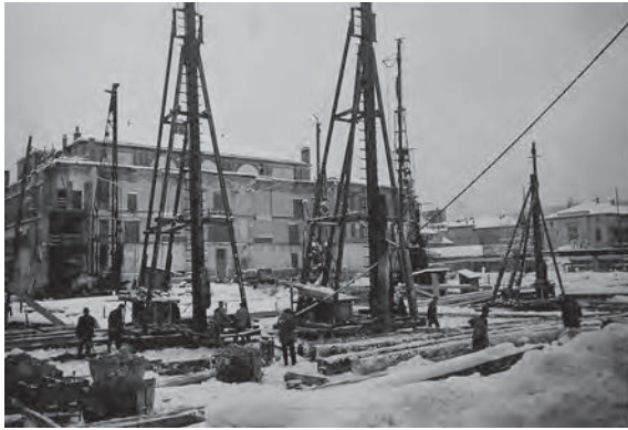
Fig. 4. Haefeli Moser Steiger Architects, Kongresshaus, Zurich, 1937–39, an archival photograph showing the timber piles being driven into the ground in 1937, and a contemporary photograph of five timber piles uncovered during excavation work in 2018. © gta Archives / ETH Zurich, Haefeli Moser Steiger, and Patrick Fleming, Conzett Bronzini Partner AG, respectively.
