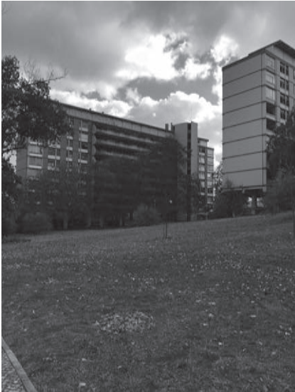
Cell A Cat.III Housing Complex in Olivais North, 1959-1964 | Cândido Palma de Melo, Artur Pires Martins. GPS: 38.775414N, 9.114904W
