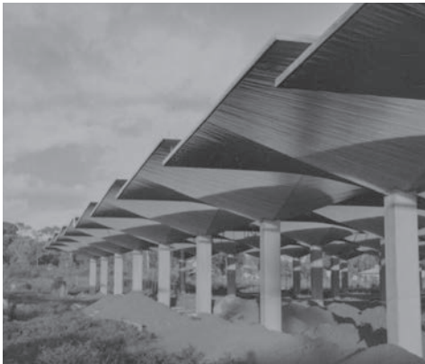
Photo of shell structures built in series for market places in 1960. The system was also used for factories. (Photo: Copy from the Castillo family photographic archive)
