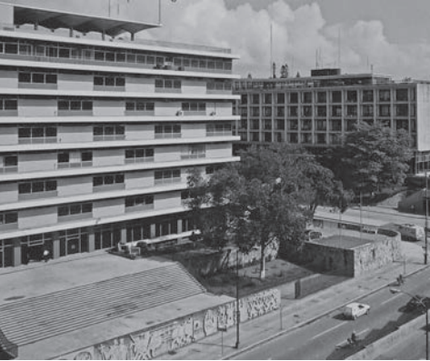
Photo of the social security building in Guatemala City, the building has a penthouse of concrete umbrellas, built in 1959. (Photo: Taken from the magazine "Galería G&T", Year 9. #26. 2006)
