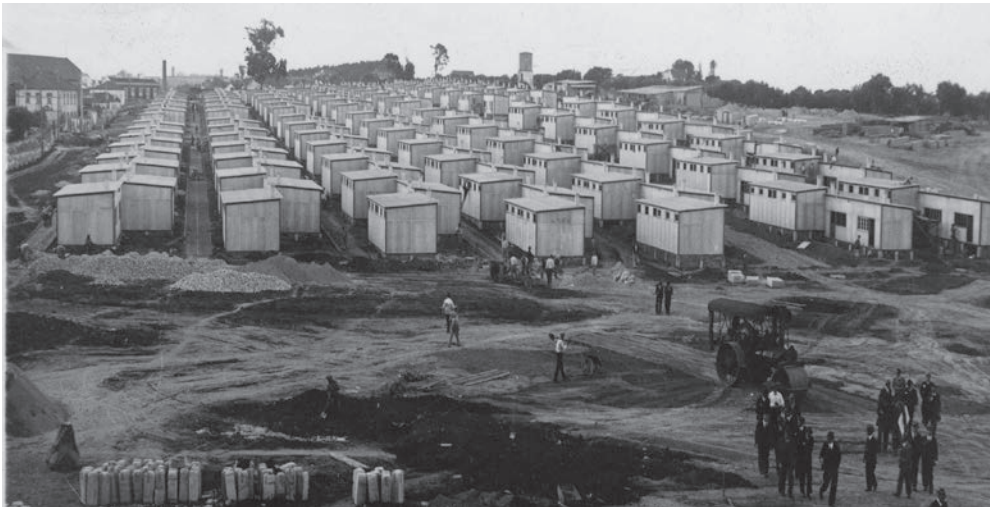
Temporary Housing Estate of Quinta da Calçada under construction. Architect Couto Martins, Lisbon 1938-39. Photography Horácio Novais. Source: Lisbon Municipal Archive.
