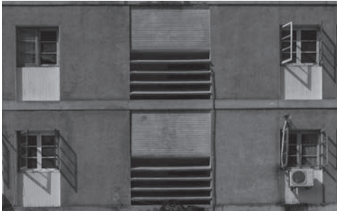
Fig. 9. Detail of the brise-soleil protecting the vertical communication core, Beira, 2020. Source: Author.
