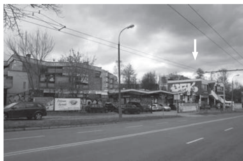
Fig. 2. "The market" pavilion complex of Słowacki Estate, Lublin, PL, a view from major street, to the right marked with an arrow – illegally enlarged pavilion. Photo: Bartłomiej Woźniak BArch, February 2020
