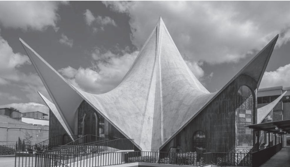
Photo of the exterior of the Shaarei Binyamin Jewish Synagogue, built in 1959. It is currently in optimum condition. (Photo: José Mata 2017)
