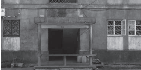
Fig. 10. Detail of the entrance framed with a concrete slab, Beira, 2020. Source: Author.
