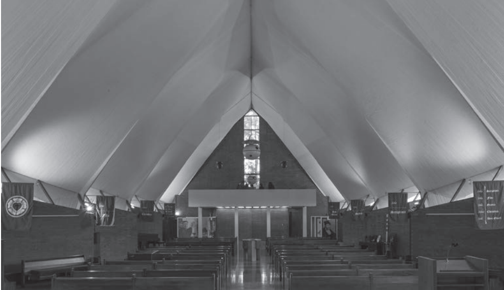
Photo of the interior of the Cristo Rey Lutheran Church, built in 1963. It is currently in optimum conditions. (Photo: José Mata, 2017)
