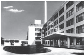
Fig 3 Tokyo Teishin Hospital (1937, Tokyo)
