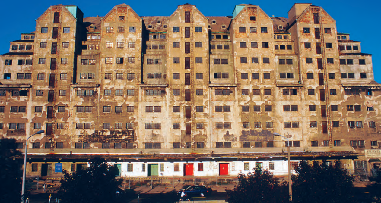
Figure 3. The warehouses were early constructions in reinforced concrete covering large areas with floor heights of only 2,40 - 2,70 m. Uta Pottgiesser.
