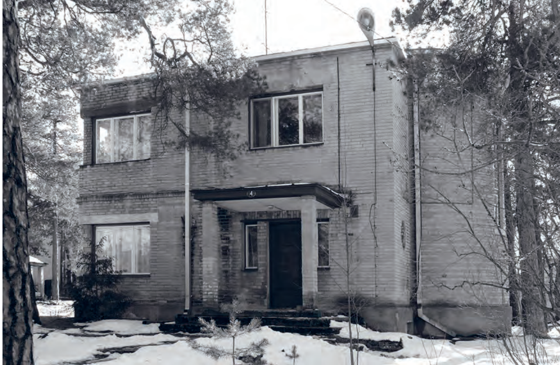
Figure 4. Calcium silicate brick in functionalism. Bruno Kadak's (the director of calcium silicate brick factory) villa in Rulli Street 4, Tallinn (1933, by E. Sacharias). Maris Suits.
