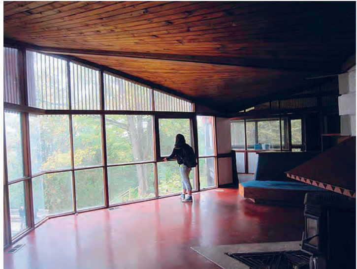
Figure 4. Wooden hyperbolic paraboloid roof and the connection with the landscape.
