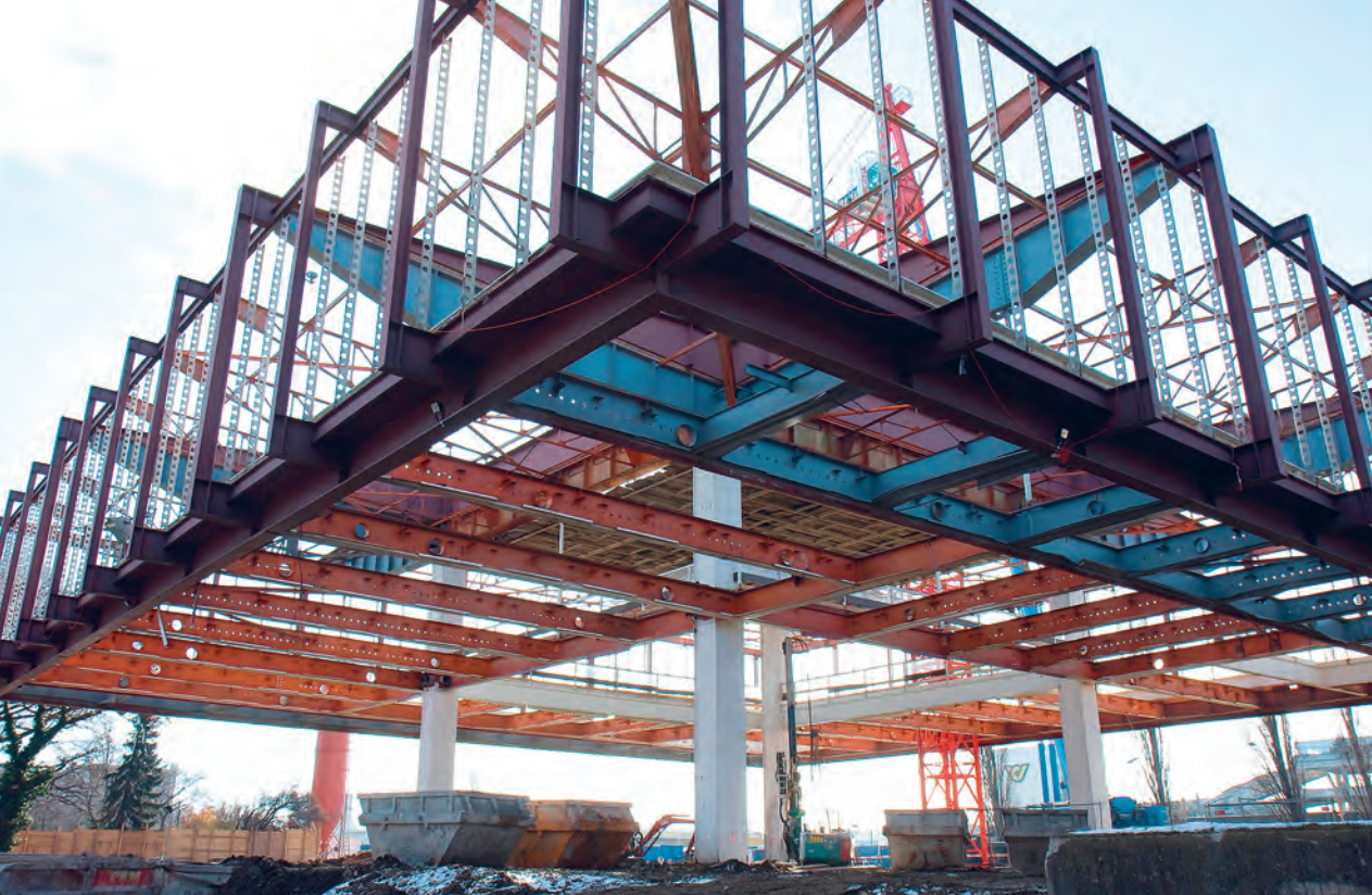
Figure 1. Steel construction of the „20er-Haus“ during refurbishment in 2009. © BDA Austria, B. Neubauer.
