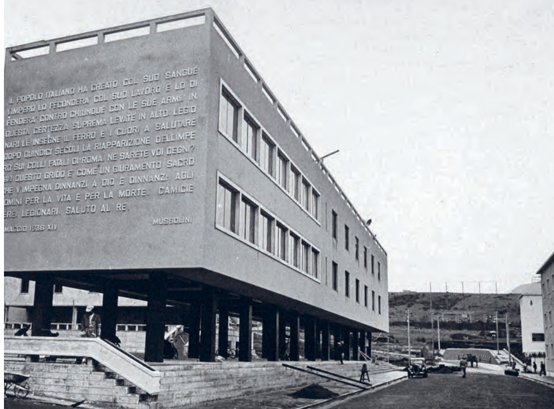
Figure 5. The office building, 1935.
