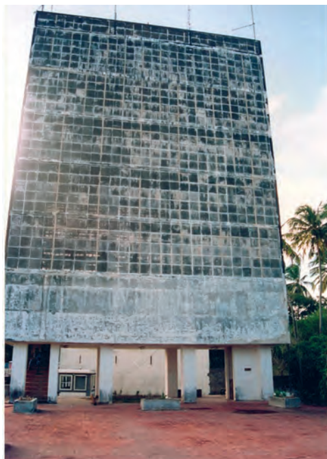
Figure 2. Olinda Water Tower before the recent restoration. Guilah Naslavsky.
