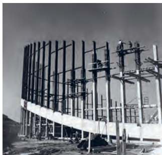
Figures 1 and 2. J S Dorton Arena, Raleigh, North Carolina.
