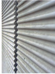
Figure 3. Gyldenrisparken after the completed renovation. Left: Note the new windows on the gables. Right: The profiling of the fibrous concrete elements on the renovated facades.
