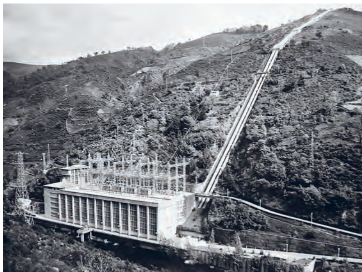
Figure 2. Vila Nova, hydroelectric power station.
