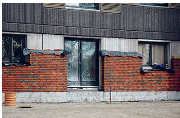
Figure 2. Vejleåparken – buildings are extra insulated, and a ‘wallpaper’ of bricks cover the architecture of the 1970s.
