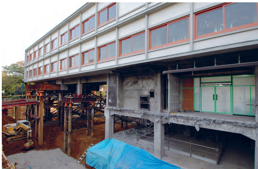
Figure 5. Extension of a new auditorium under construction.
