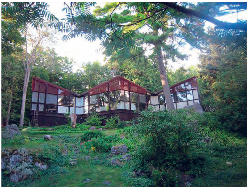
Figure 1. Exterior view of the Strutt House, sensitively integrated into their natural environment.
