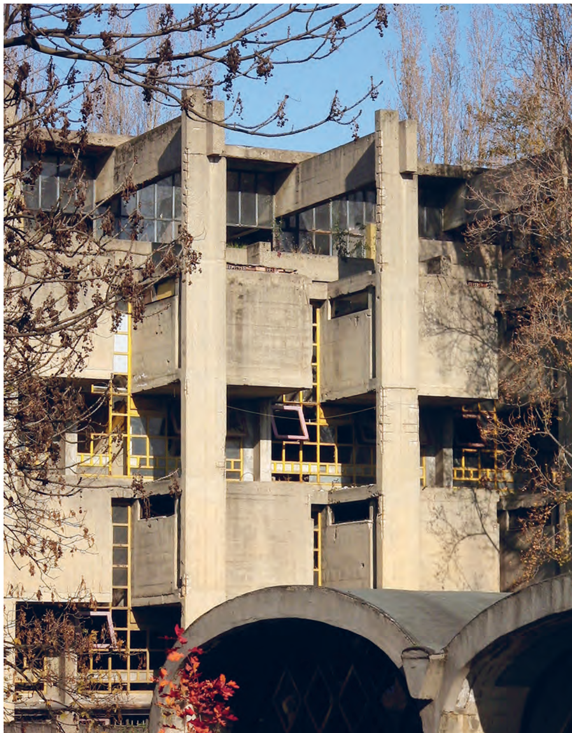
Figure 1. External view of the Residential Block.
