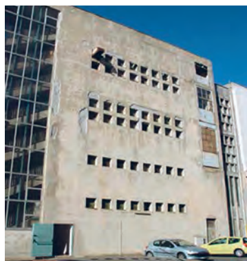
Figure 6. Building “B” before demolition (2009).
