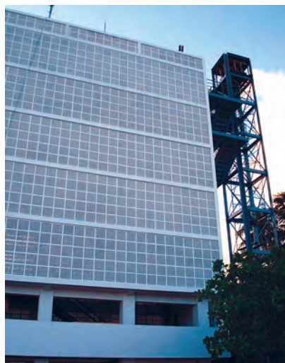
Figure 3. Olinda Water Tower after the recent restoration. Eduardo Pinto.
