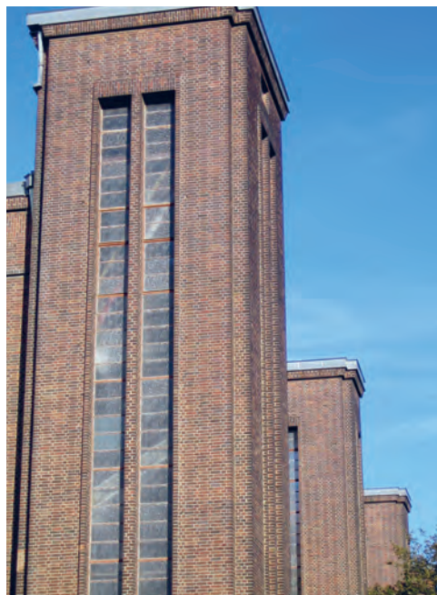
Figure 2. The typical decorative brick facade of the early 20th century is combined with an industrial glazing system of the late 19th century; envelope of a modern energy plant. Uta Pottgiesser.
