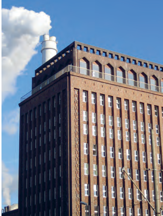
Figure 1. The administration building of Kraftwerk Klingenberg (1925-26) has large vertical brick columns but shows horizontal separations at floor level with a perforated facade for the office functions. Uta Pottgiesser.
