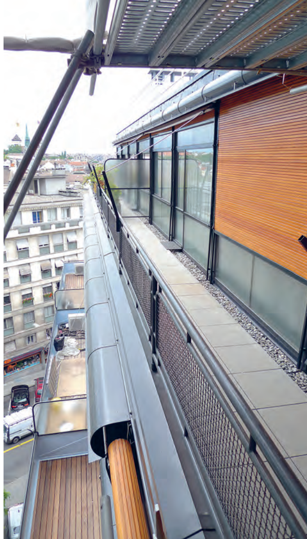
Figure 4. After restoration and improvements. Carmen Reolon, Private Photographic Archive, 2009.
