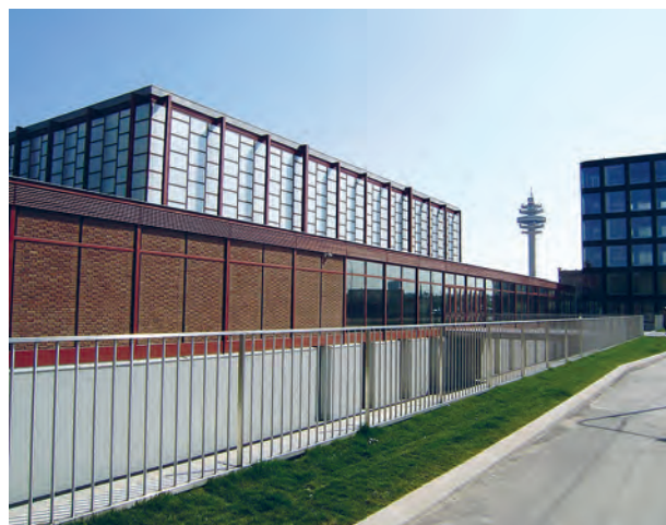
Figure 5. The original curtain wall facade of the former Hoffmann-La-Roche building. Today „Hotel Daniel“, after restoration in 2012. © BDA Austria, W. H. Salcher.
