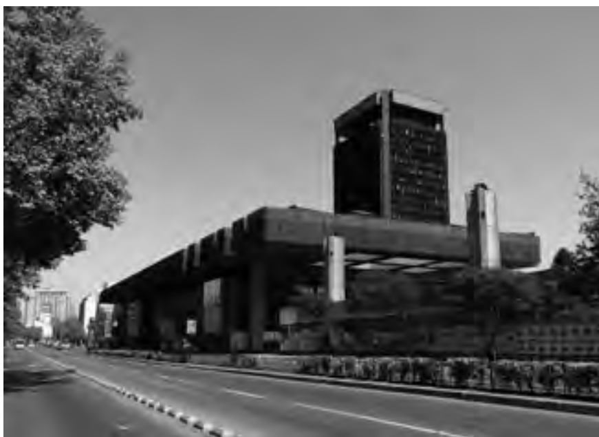
FIGURE 2. José Covacevic, Hugo Gaggero, Juan Echenique, José Medina, Sergio González Espinoza (1972); Cristián Fernández and Lateral (2005), UNCTAD III Building, Centro Cultural GAM, Santiago, Chile. View of the building in its present state. © Maximiano Atria.
