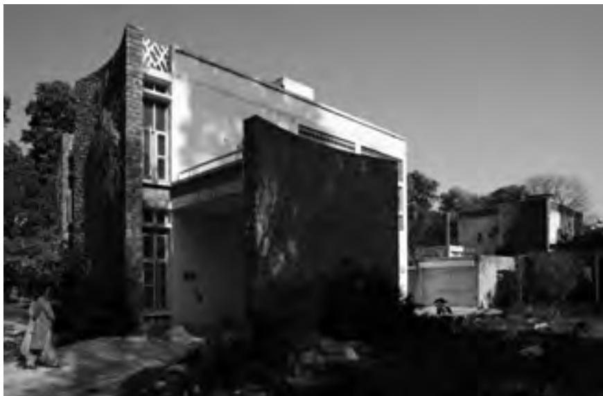
FIGURE 1. Pierre Jeanneret, Own House, Chandigarh, India, house and its garden setting. © Franco Panzini, 2008.
