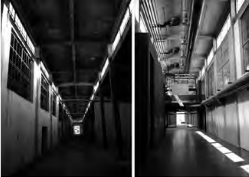
FIGURE 4. Burak Asiliskender and Nilüfer Baturayoglu Yöney, Abdullah Gül University Sümer Campus, Restoration and Adaptive Reuse Project for the Great Storehouse , interior views, 2015 (left) and 2016 (right). © Burak Asiliskender.
