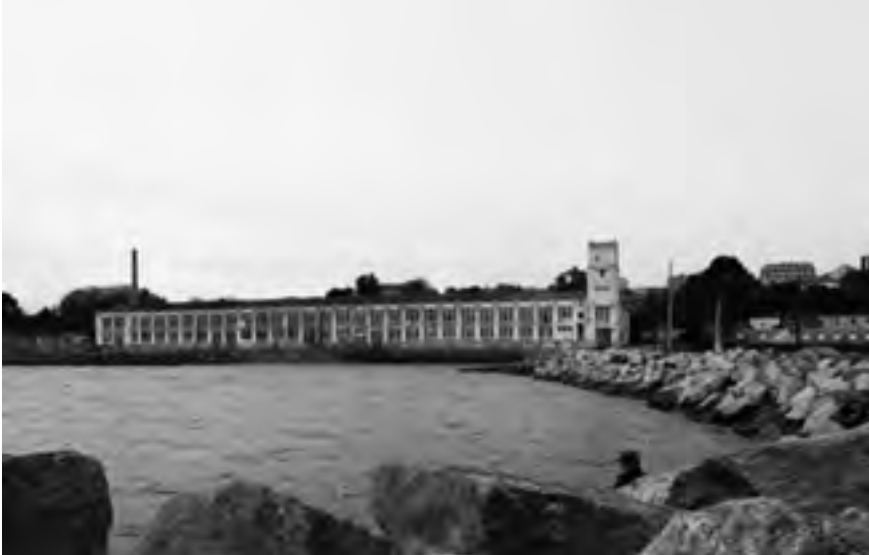
FIGURE 1. Massó Canning Factory, Cangas do Morrazo, Spain, the main factory building (left) and the former facility building (right), which became O Salgueirón squatted autonomous social centre from 2010 to 2012. © Eva Maria Hierzer, 2010.
