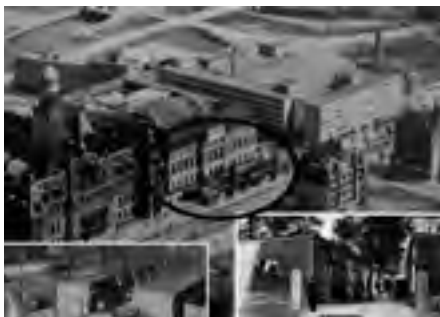
FIGURE 2. Temporary shops in the bombed city centre during the German occupation years 1940-1945. © Municipal archives de Rotterdam.
