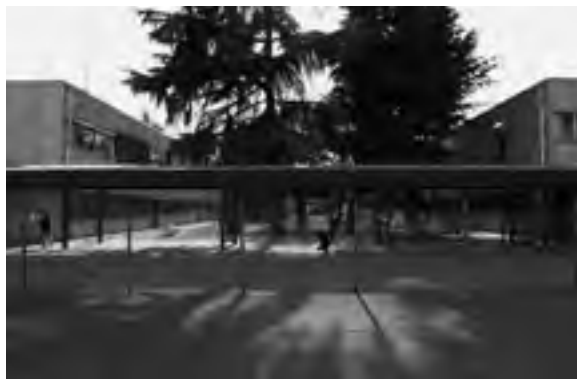
FIGURE 4. Studio Architetti Valle, school to Chirignago, Venezia © IC “Cristoforo Colombo”, 2016.
