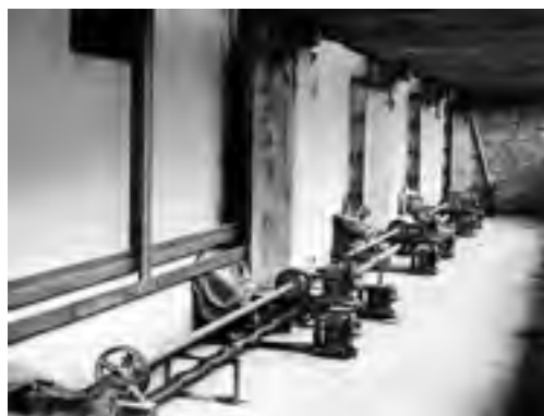
FIGURE 3. Mario Labò, Giorgio Olcese, Luciano Grossi Bianchi and Cesare Fera, The Museum of Japanese Art “Edoardo Chiossone”, Genoa, Italy, 1949-1972. The steel frames of the windows and the electrical mechanism for their movement (defective almost from the beginning). © Archive of Public Works, Municipality of Genoa.
