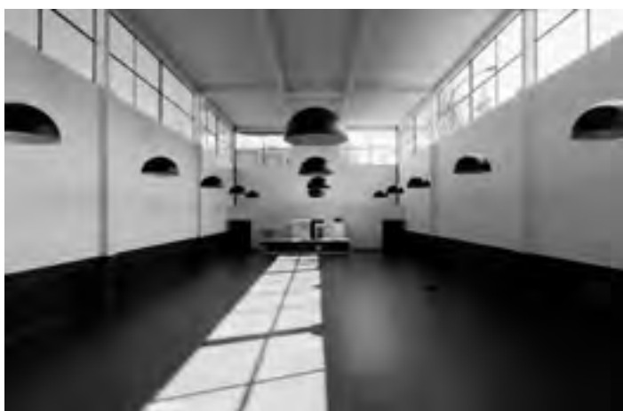
FIGURE 4. André Lurçat, Karl-Marx school, Villejuif, France, 1933. Gymnasium after restoration and reuse as a school-restaurant for 120 seats. © Niels Stoltenborg, 2012.
