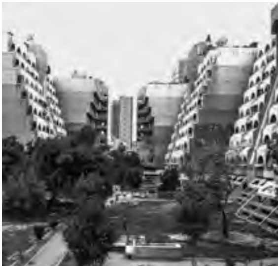
FIGURE 3. Arthur Erickson, Al-Sawaber, Kuwait, weathering of the Al-Sawaber complex showing tenant balcony expansions. © Asseel Al-Ragam, 2016.
