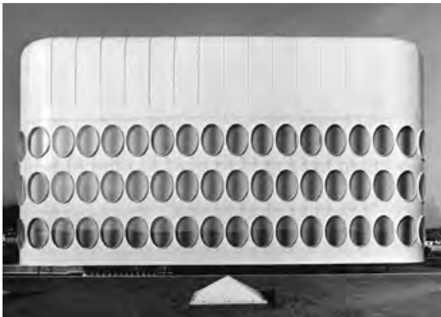
FIGURE 4. Angelo Mangiarotti, Snaidero Factory, Majano, Italy, 1971-1978. Office Building © Trust Fondazione Angelo Mangiarotti Milano .
