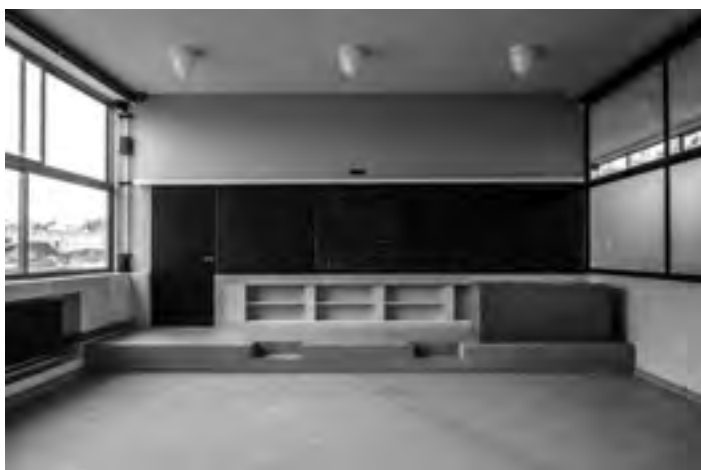
FIGURE 3. André Lurçat, Karl-Marx school, Villejuif, France, 1933. Classroom after restoration. © Priska Schmückle von Minckwitz, 2003.
