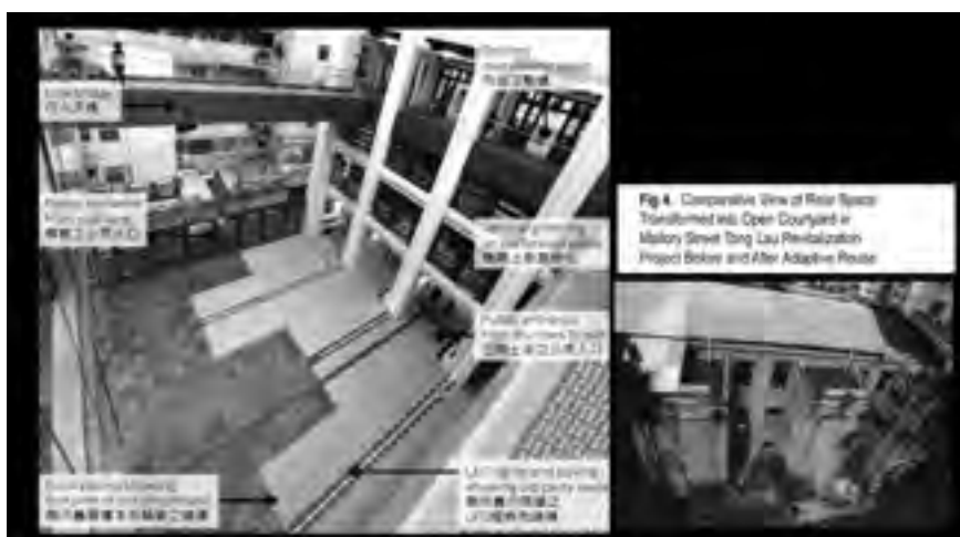
FIGURE 4. Comparative view of rear space transformed into open courtyard in Mallory Street Tong Lau revitalization project before and after adaptive reuse. © Edward Leung.
