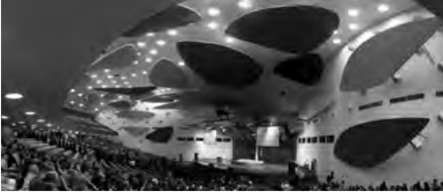
FIGURE 1. The Aula Magna lecture theatre shows integration between architecture, technology and art. The features of the ceiling, commonly called “the clouds”, were designed by the artist Alexander Calder for acoustical purposes. © Adriana Salas, 2013.
