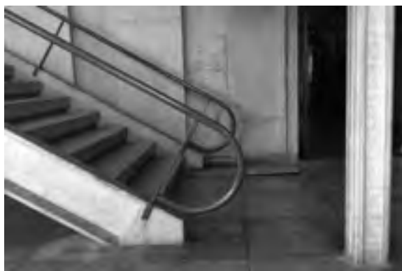
FIGURE 4. João Filgueiras Lima, Modular school at Faculty of Architecture – UFBA, Salvador, Brazil, 1988. © Ceila Cardoso, 2015.
