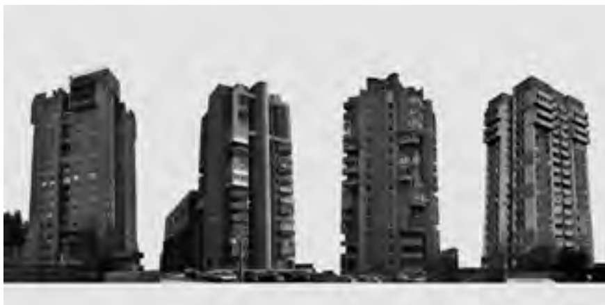
FIGURE 1. From the left: Česlovas Mazūras, 16-storey tower block in Lazdynai district, Vilnius, 1978-85; Edmundas Stasiulis, 16-storey tower block in the Konstitucijos Ave., Vilnius, 1983; Bronius Krūminis, Danas Ruseckas, 16-storey tower block in Šeškinė district, Vilnius, 1983; Česlovas Mazūras, 16-storey tower block in Justiniškės district, Vilnius, 1980. © Aušra Černauskienė, 2013.
