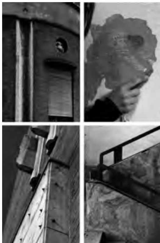
FIGURE 1. Arnaldo Fuzzi, Casa del Fascio , Predappio, Italy, 1934-1937. From top left: reinforced concrete kerb; association of traditional materials and industrially-produced materials in a mixed vertical structure; Stimip horizontal structure with unidirectional trend; Stimip horizontal structure with bidirectional trend. © Giulia Favaretto, 2015.
