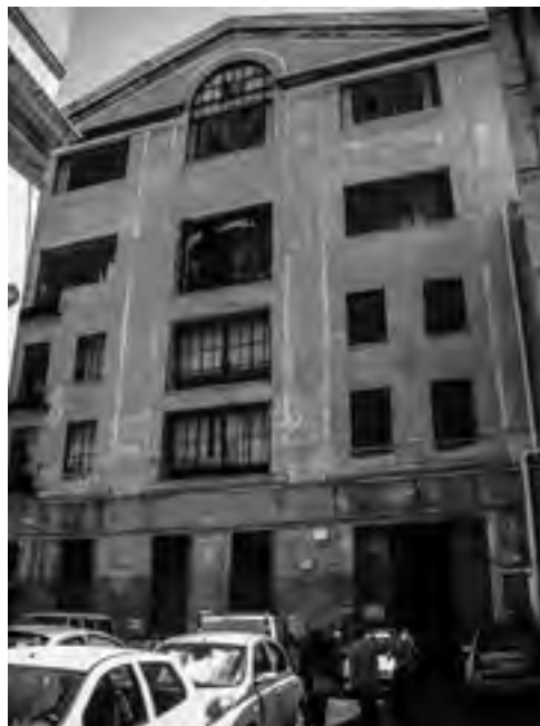
FIGURE 2. The inner courtyard and the building site of the Rome Opera Theater Laboratory of scenography. © Alessandra Marin, 2015.
