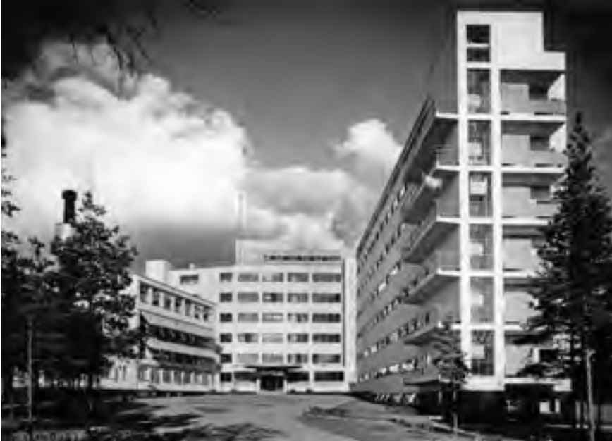
FIGURE 1. Alvar Aalto, Paimio Sanatorium, Paimio, Finland. The main entrance of the completed Paimio Sanatorium in 1933. © Alvar Aalto Museum, Photo Archive 50-003-215, Weilin, 1933.
