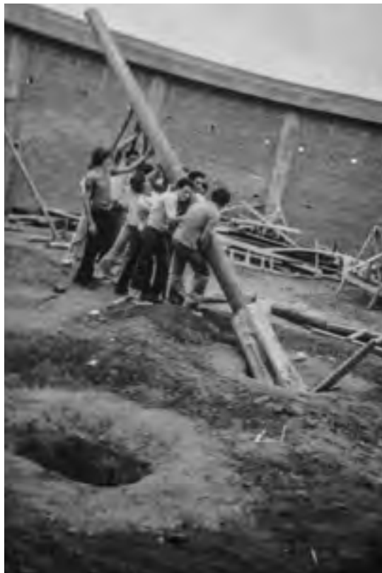
FIGURE 2. Lina Bo Bardi, Construction Divino Espírito Santo do Cerrado Church, Uberlândia, Brazil, 1980. © Courtesy of Community Jaraguá Neighbourhood.
