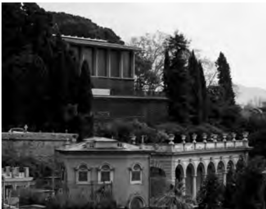
FIGURE 1. Mario Labò, Giorgio Olcese, Luciano Grossi Bianchi and Cesare Fera, The Museum of Japanese Art "Edoardo Chiossone", Genoa, Italy, 1949-1972. View of the south façade. The museum was built after WWII demolition of a small villa in the urban park. © Luca Pedrazzi, 2013.
