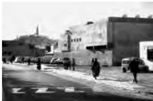
FIGURE 3. André Ravéreau, Post office of Ghardaïa, M'Zab valley, Algeria, 1966-67. © Manuelle Roche/ADAGP, Ravéreau's private archive, Manuelle Roche photographer.
