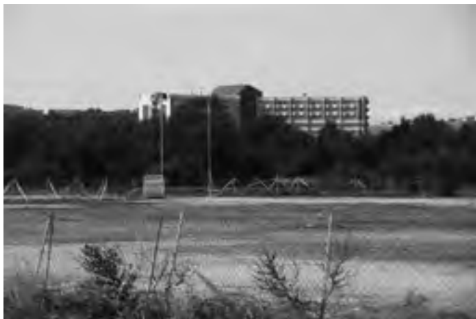
FIGURE 2. Jet Residence, Portorecanati (MC), Italy, 1970s. The structure situated in an isolated portion of Portorecanati city, is now underexploited, its volume and its dimension confirm the choice of an urban macroscale for the mass tourism accommodations. © Sara Cipolletti, 2015.
