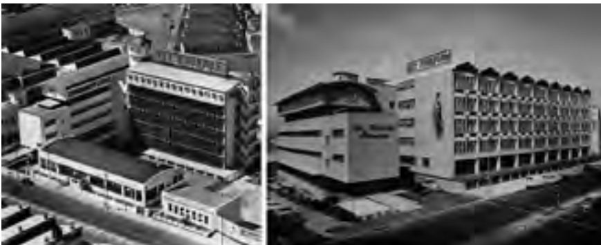
FIGURE 1. Andrews and Niegeman, Turok, Rex Trueform factory, Salt River Cape Town, South Africa, 1947-1963. © Architect & Builder, 1965 right, Supplement to the Buyer, 1947, left.
