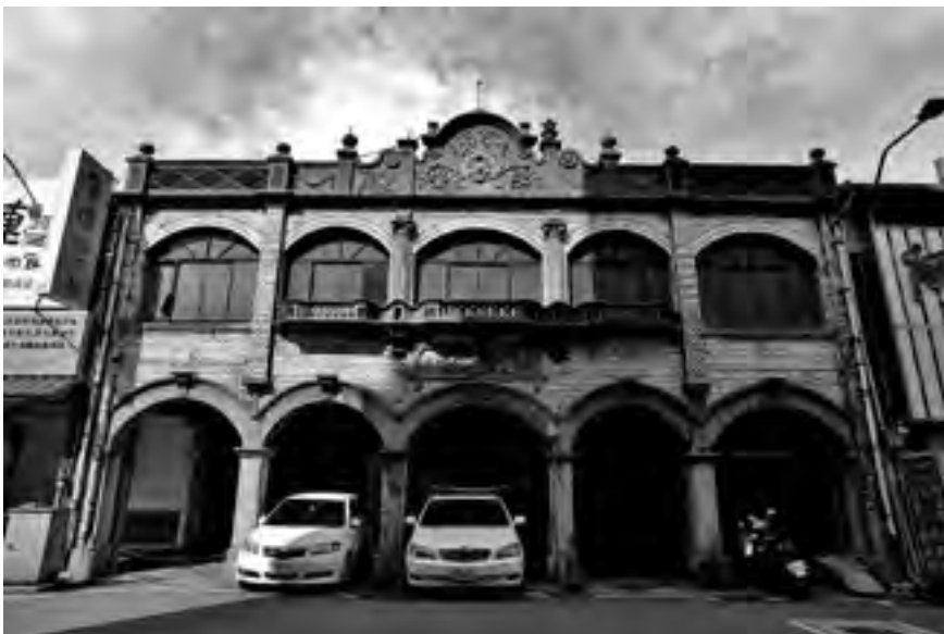
FIGURE 1. Present-day façade view of the B.S. House & Heritage. © Yuta Chou, 2014.
