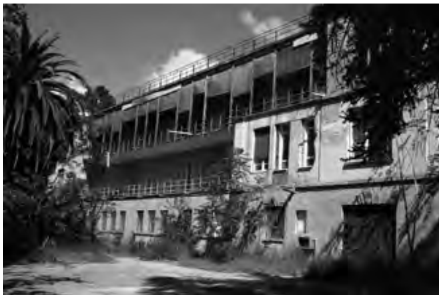
FIGURE 4. The Dubini sanatorium in a state of abandonment and the damage to its façade. © Tiziana Basiricò, Antonio Cottone.
