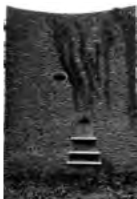
FIGURE 2. Pierre Jeanneret, Own House, Chandigarh, India, the stone wall, inset arch window and oval window. Elements of the rear façade. © Franco Panzini, 2008.
