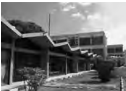
FIGURE 3. Ahmet Vural Behaeddin, Lefkosa Turkish Boarding School for Girls, Nicosia, Cyprus, 1960-63. Vertical shading devices on the east façade and concrete lattice for vertical circulations. © Sevil Aydinlik.
