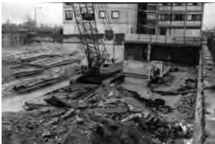
FIGURE 3. Deck between parking level and pedestrian level is being renewed after less than ten years of tear. © Forstadmuseet, 1978.
