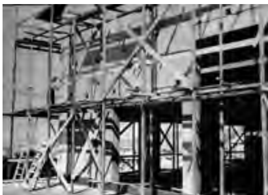
FIGURE 2. Mario Labò, Giorgio Olcese, Luciano Grossi Bianchi and Cesare Fera, The Museum of Japanese Art “Edoardo Chiossone”, Genoa, Italy, 1949-1972. The construction of the reinforced concrete structure and external brickwork. View of the south-east façade. © Archive of Public Works, Municipality of Genoa.
