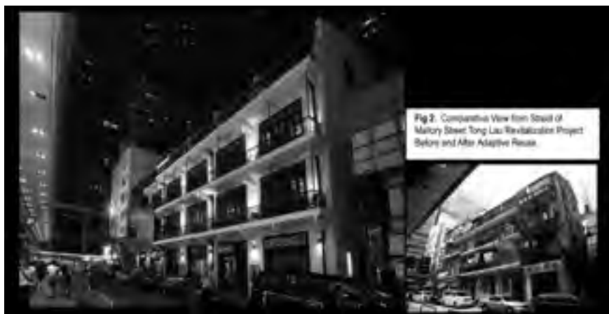
FIGURE 2. Comparative view from street of Mallory Street Tong Lau revitalization project before and after adaptive reuse. © Edward Leung.
