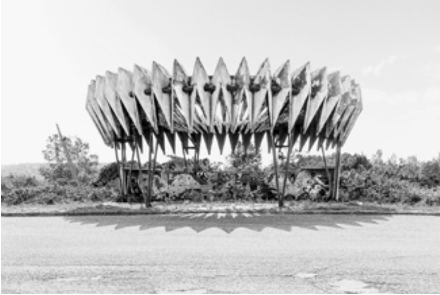
FIGURE 4. Architect unknown, bus stop, Pitsunda, Disputed region of Abkhazia. © Christopher Herwig, 2015.
