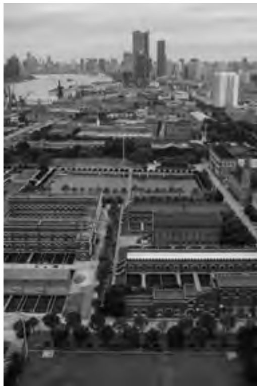
FIGURE 4. Yangshupu Water Plant. © Songsong Li, Subin Xu.
