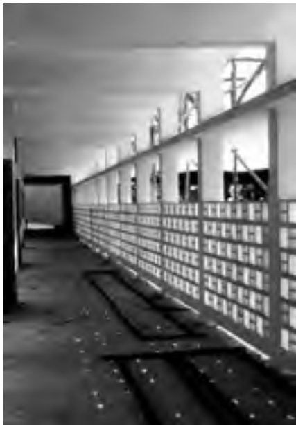
FIGURE 3. Silva Dias and Jacinto, School Complex, Saurimo, Angola, 1959-1960. Construction works. © Francisco Silva Dias and Antonieta Jacinto Archive, 1960.
