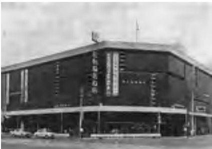
FIGURE 1. Kenji Mitsuyoshi, Maruya department store, Kagoshima, Japan, 1961, after completion of original construction. Taken in 1961. © Maruyahonsha House journal, Maruyahonsha Co., Ltd.
