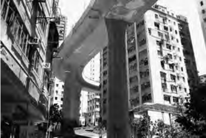
FIGURE 1. Hill Road Viaduct, Sai Ying Pun, Hong Kong. © Peter Ferretto, 2015.
