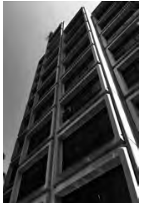
FIGURE 3. Tao Gofers, Sirius Towers, Sydney, Australia, 1978, the interlocking modular concrete façade units. © Leigh Hanekom.
