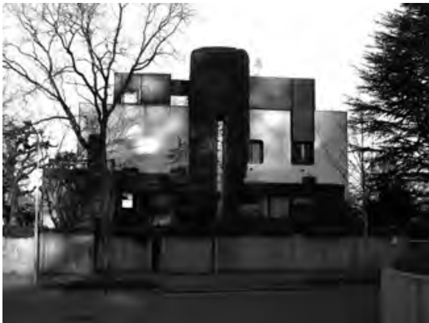
FIGURE 1. Carlo Scarpa, Casa Zentner , Zurich, Switzerland, 1965-67. Façade along Aurora Strasse. © Giacinta Jean, 2015.
