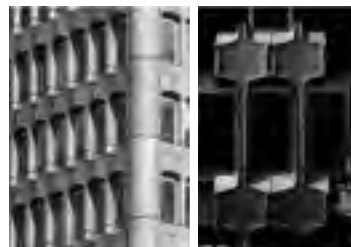
FIGURE 4. Eugène Beaudouin, Alberto Camenzind, Pier Luigi Nervi, International Labour Organisation building, Geneva, Switzerland, 1965-72. © Giulia Marino, 2014 (right), Camenzind Archives, Zurich (left).
