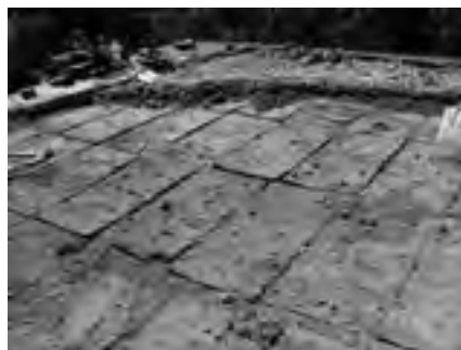
FIGURE 4. Emil Lange, detached house of the WuWA estate, Wrocław, Poland, flat roof original insulation Torfoleum plates. © Jadwiga Urbanik, 2014.
