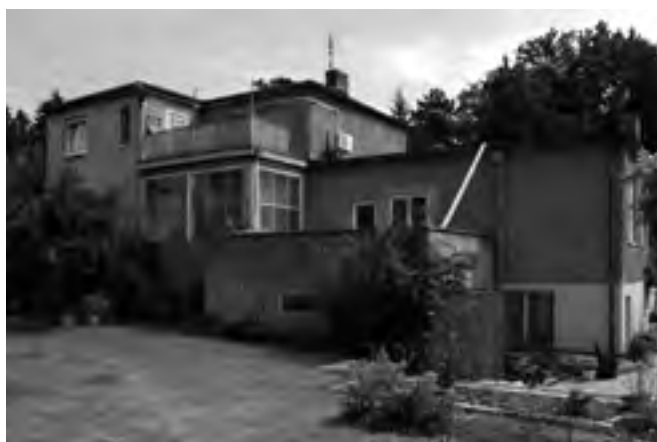
FIGURE 2. Emil Lange, detached house of the WuWA estate, Wrocław, Poland. Garden view. © Jadwiga Urbanik, 2014.
