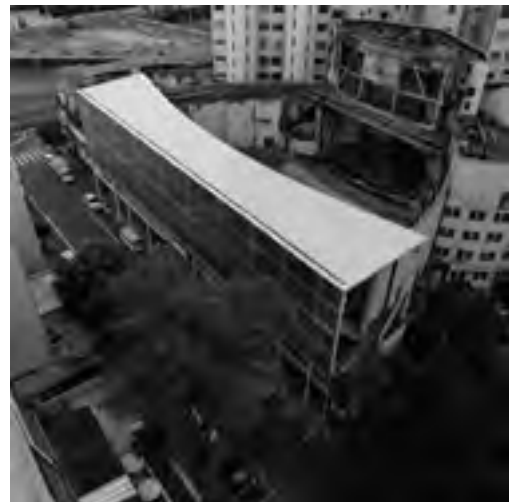
FIGURE 2. The theatre after the fire that destroyed it. The steel structure was built to prevent the collapse of the front mural. © Nelson Kon.
