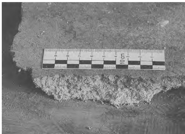
Fig. 4a: Woodcement-magnesite-flooring. NARKOMFIN-Commune House. Moscow 1928–30. Photo 2009.
