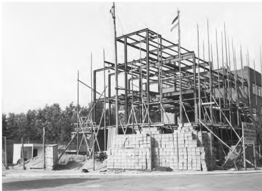
10. The building of the modern skeleton of the Van der Leeuw House, Rotterdam 1928 (Photo source: unknown).
