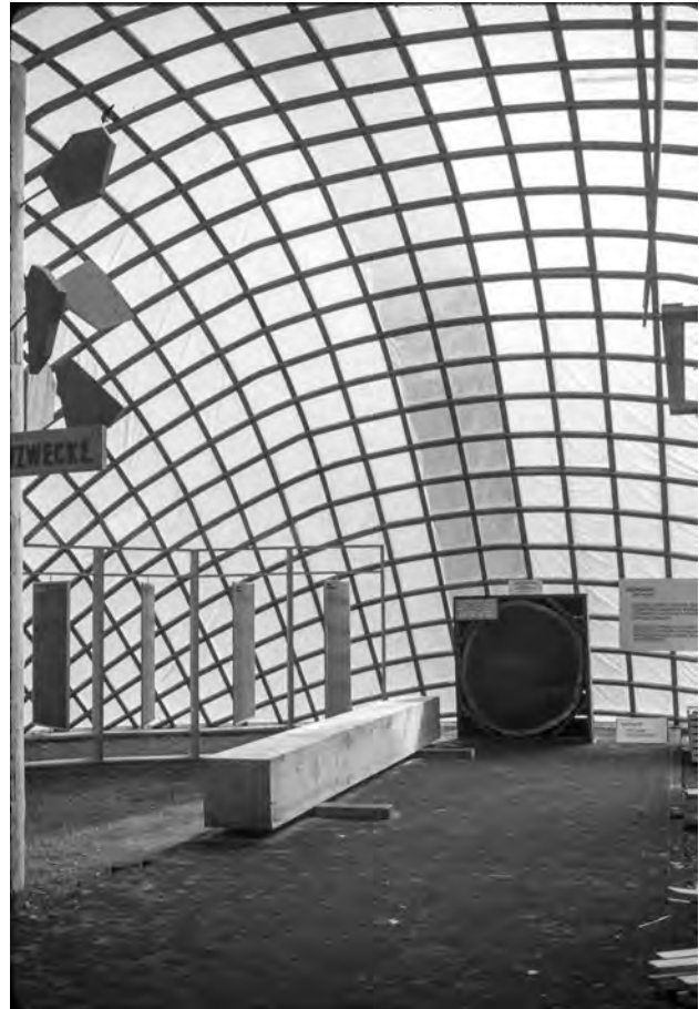
Fig. 4: Essen DeuBau. Second grid shell shaped on pneumatic structure. (Photo Frei Otto 1962).
