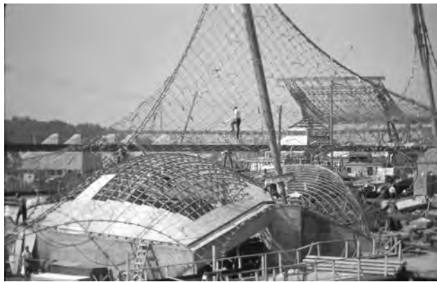
Fig. 5: Montreal Expo 67 Construction of cable net. In foreground grid shells covering the auditorium (Photo Frei Otto 1966)
