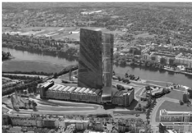
Figure 14: Design of the headquarter of the European Central Bank (ECB) in Frankfurt/Main by Coop Himmelb(l)au, 2008. The refurbished Grossmarkthalle has been added by a 200 m twin office tower and other additions.
