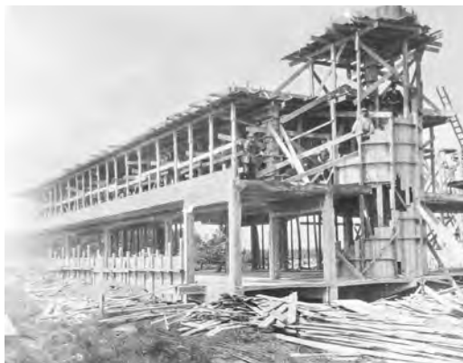
Fig. 6c: Detail of 6a with tapering floors between high beams. The big console beam to the right, carries one of the spiral stairs.
