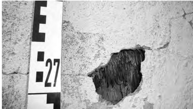
Fig. 12: Plastered Kamyshit -matting. Prototype of an external thermal insulation composite system. NARKOMFIN Commune House. Moscow 1928–30. Photo 2009.
