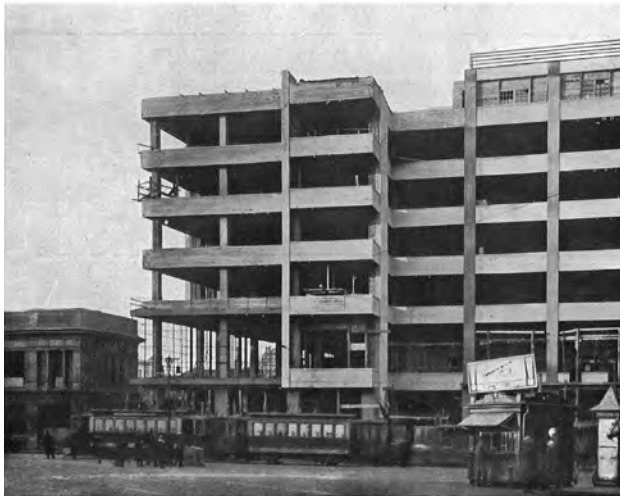
Fig. 2a: GOSTORG - Ministry of Trade. Concrete-skeleton. Moscow 1925–27. Credit: El Lissitzky (1930), Abb.75.
