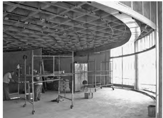
Fig.2b: Hall with waffle slab and flat gypsum low-ceiling. Photo: Danilo Matoso (during renewal in 2002).
