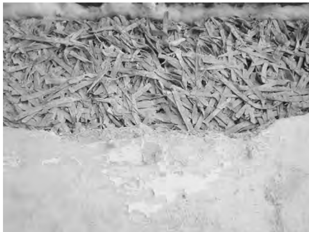
Fig. 4: Fibrolit-panels as interior insulation. NARKOMFIN-Commune House. Moscow 1928–30. Photo 2007.
