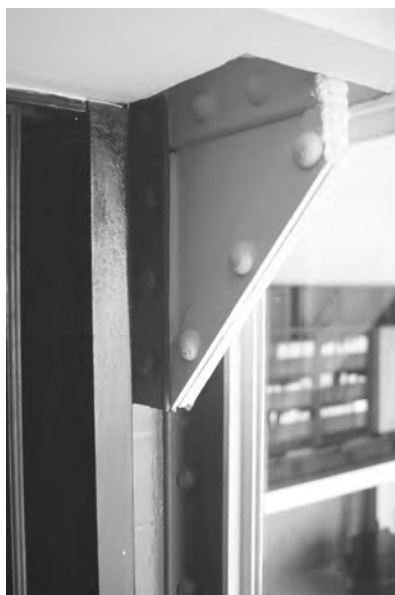
Fig. 12: Console of one of the columns (Photo Jan Molema 2012).
