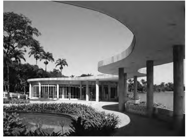
Fig.2: Casa do Baile, Belo Horizonte, 1940. Oscar Niemeyer, Architecture. Albino Froufe, Structural Engineering. Marquee with flat ceiling and inverted beams. Photo: Alexandre Brasil.
