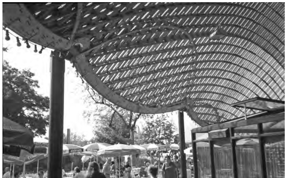
Fig. 9: Mannheim Multihalle wooden grid shell. The picture shows border divisions of the grid shell held by a cable between standing posts (Photo Frei Otto 1975)
