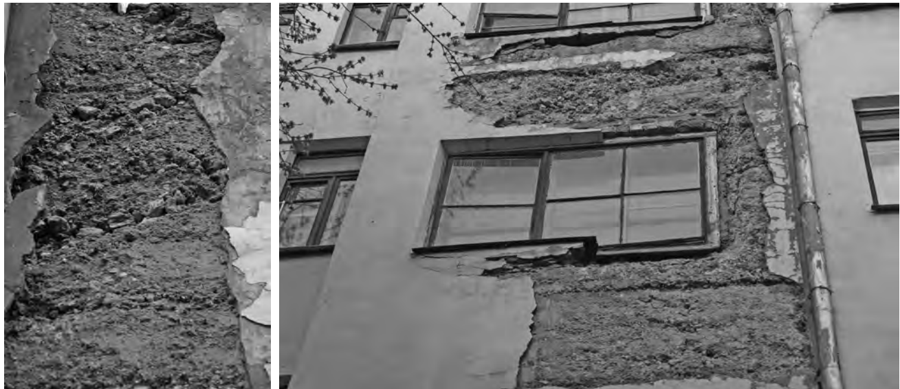
Fig. 3: Kossel-slag concrete, named after the constructor Paul Kossel from Bremen, Germany. With his assistance a German-Russian construction trust RUSGERSTROY built the dormitory of the Red Professors on Pirogovskaia Street in Moscow 1925–28. The same Kossel-slag concrete was used in different mixtures for the houses of Johannes Pieter Oud in the Weißenhof-settlement in Stuttgart in 1927. Photo 2005.
