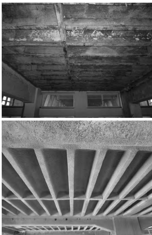
Figure 16: Ribbed ceiling, before and after refurbishment.
