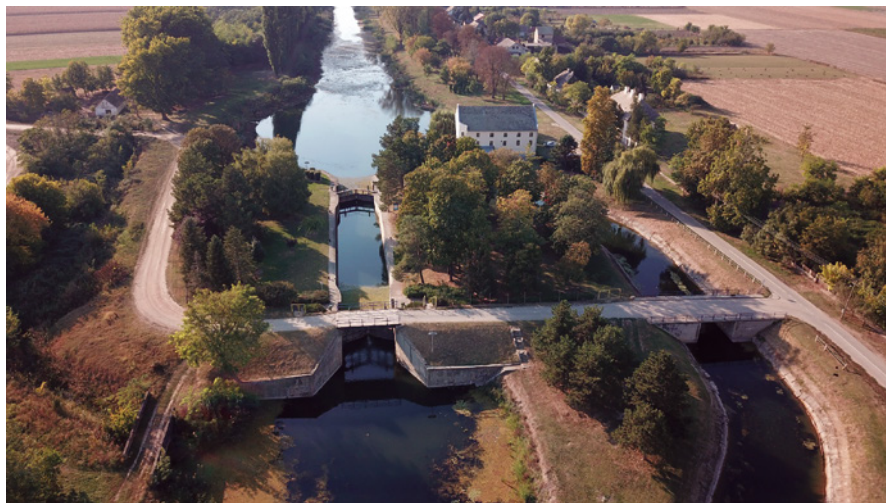
Figure 157 The dam on the Tisa River of the Hydro System Danube-Tisa- Danube. © Vode Vojvodine public company.
