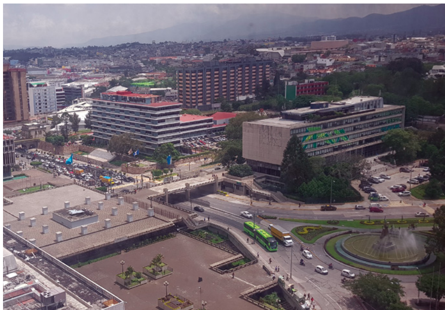
Figure 34 View of the Guatemala Civic Centre walkways and Seventh Avenue. © Sonia Fuentes, 2019.
