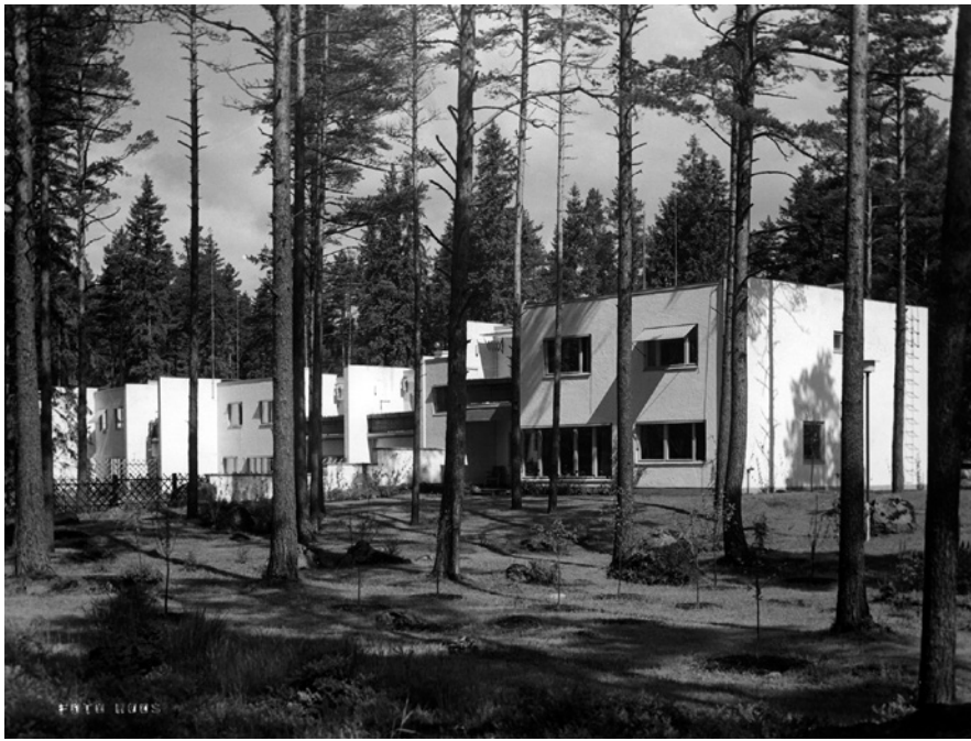
Figure 31 The engineers' row house, as well as the other housing, was carefully situated according to the topography of the landscape and orientation, as seen in this photograph from the 1930s. Privacy to the gardens was provided by the shape of the building and the fan-shaped opening towards the south-west. © Alvar Aalto Museum, Foto Roos, sign. 81-002-019.
