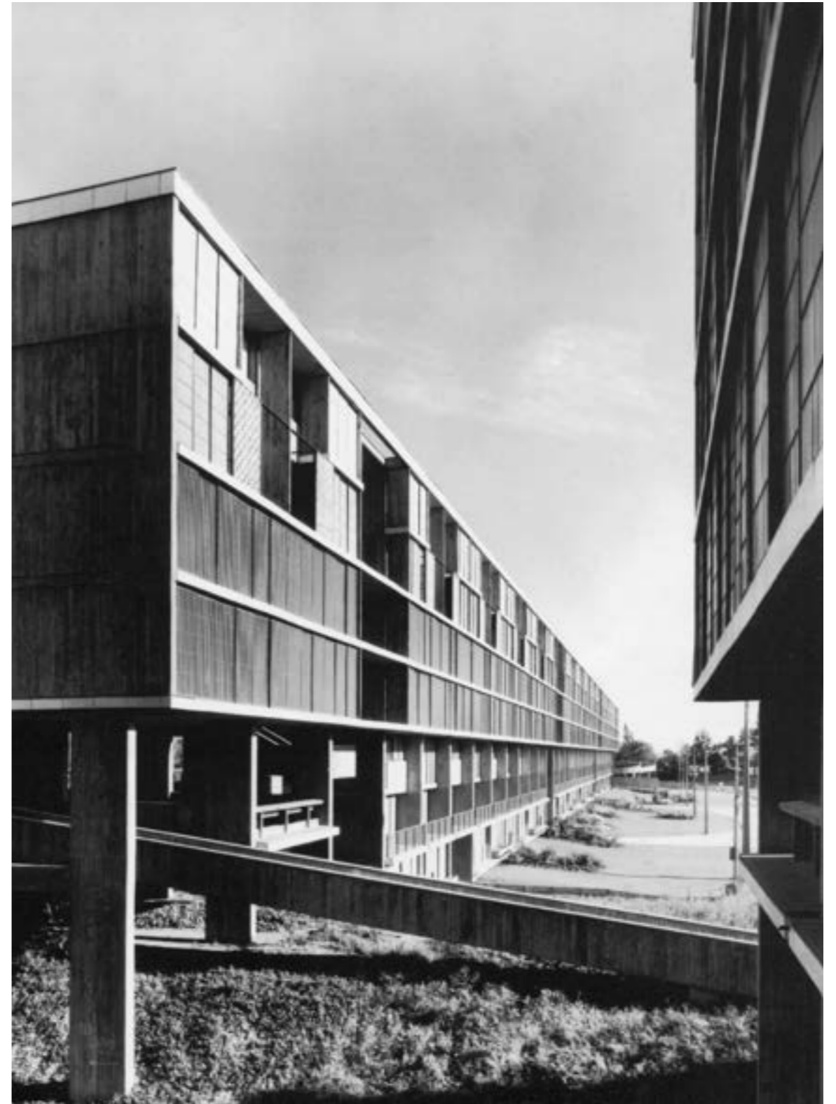
Portales Neighborhood Unity. Bresciani, Valdés, Castillo, Huidobro, 1953-1967 Photo René Combeau, Original photo archive of FADEU - PUC
