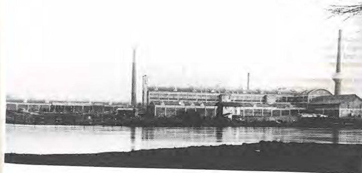
Division II during construction in 1912, view from the south. photo: Social Historical Centre for Limburg, Maastricht.
