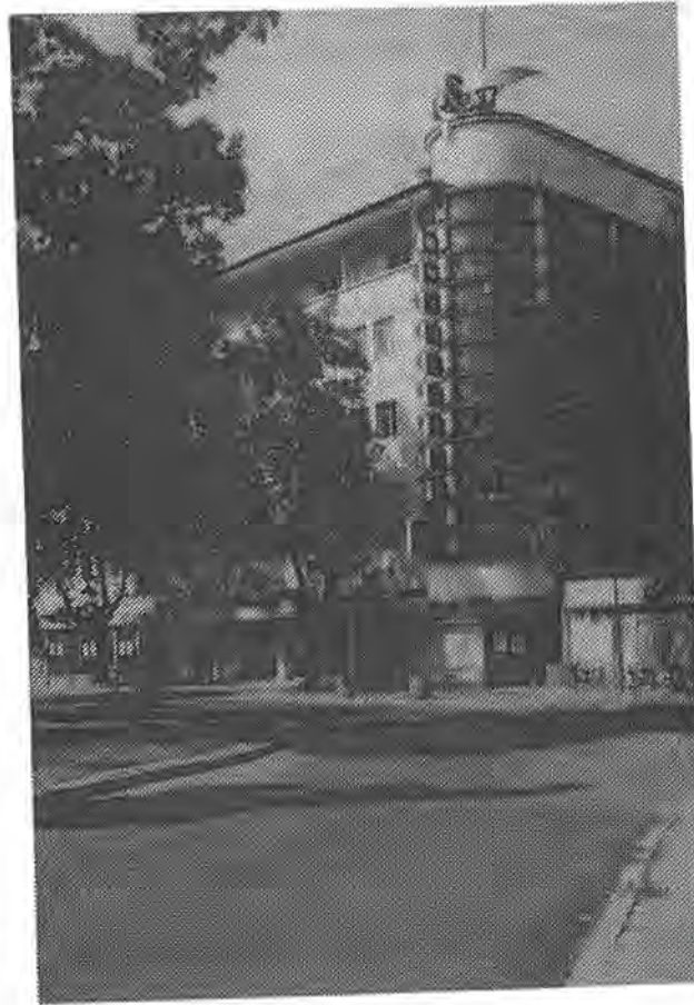
The Picture Cinema "Osvobozhdenie" in Sofia Architect A. Delibashev, 1938
