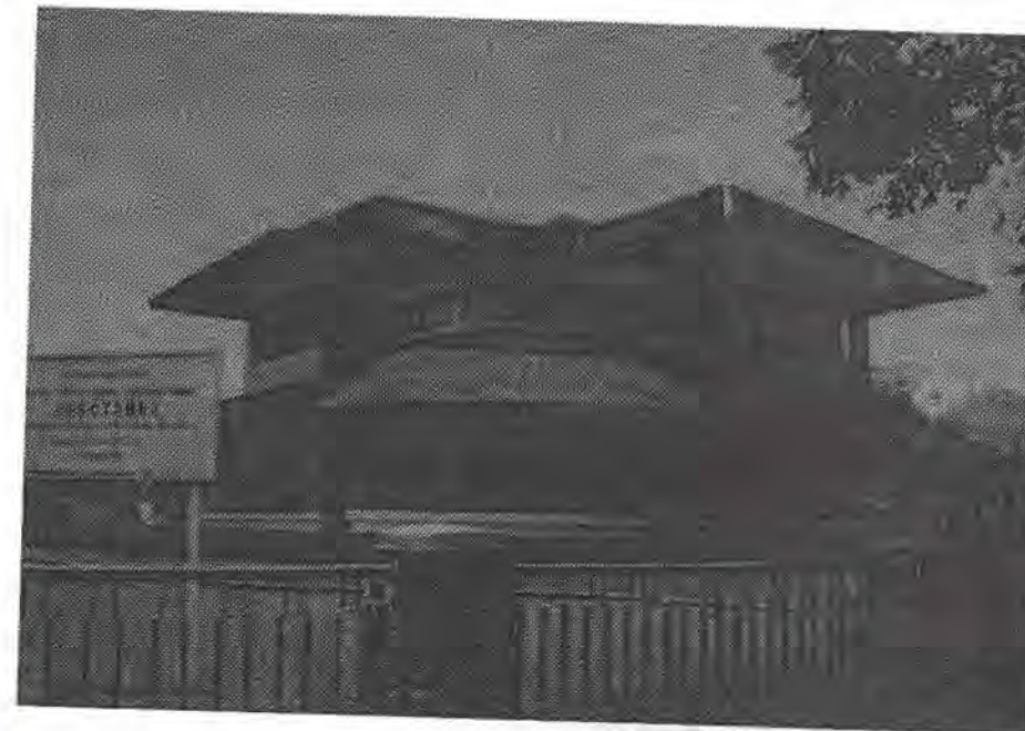
Bandung: large roof overhangs and ample ventilation, mark the luxurious houses in the spacious residential district where the Europeans lived. photo: R. Gill
