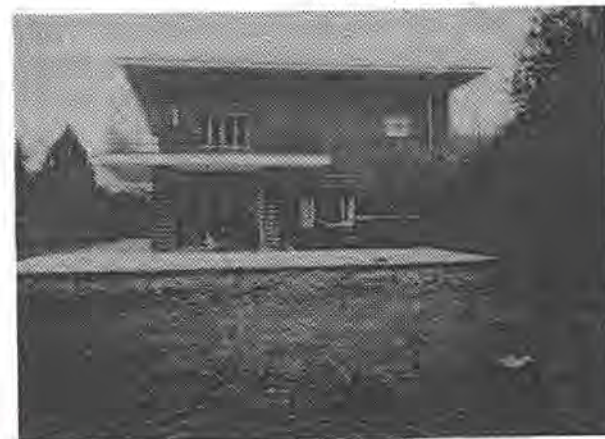
Soest, Villa Jahn Architect Bruno Paul, 1929-30 photo: Department of Conservation Westfalia (E. Grunsky)
