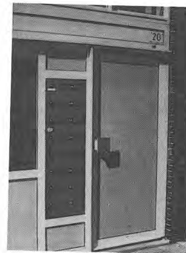
Landlust entrance at the street side, after renovation with synthetic profiles dominating the smooth facade.
