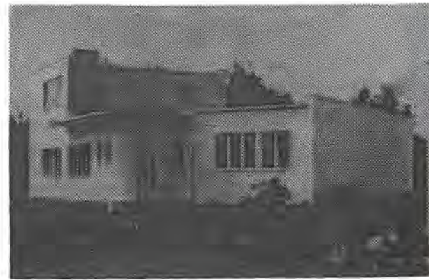
Ludwig Moshamer: One family house Breslau WUWA Exhibition 1929 Ostdeutsch Bau-Zeitung, Breslau 1929, p. 445
