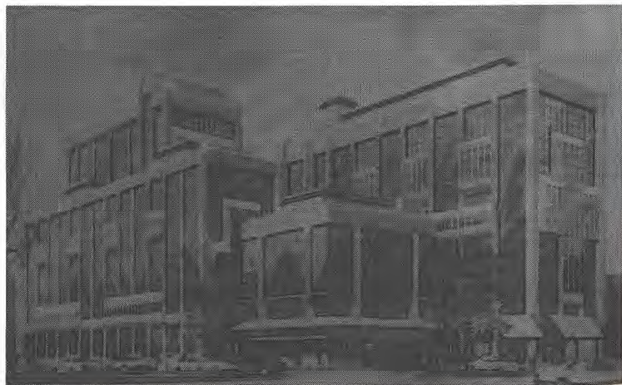
Alexander Fleming House, Ernö Goldfinger 1960, with proposed rainscreen overcladding by Fairhurst Architects 1988
