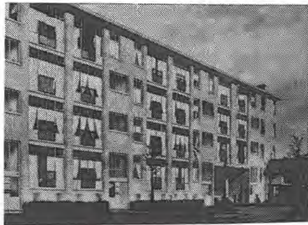
Landlust streetside, original situation with thin steel profiles, doors and transparent "french balconies" in front of the big windows.
