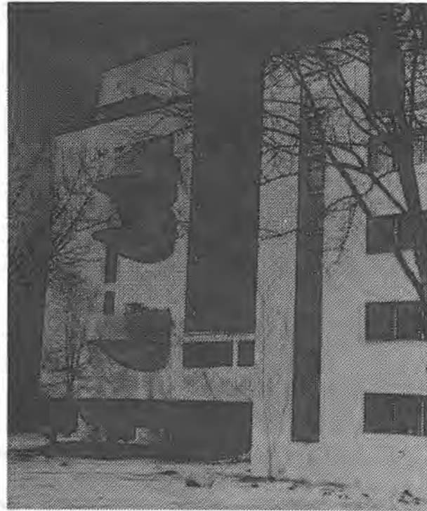
Ginzburg & Milinis: Narkomfin housing complex, Moscow, 1928-30, with residential wing, left and communal facilities, right (photo soon after completion)
