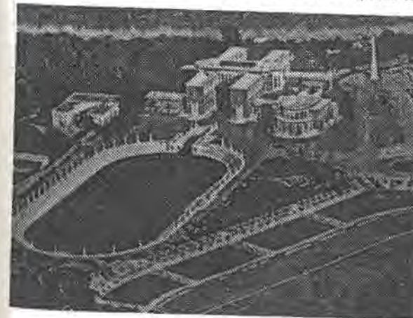
The buildings of the Accademia Fascista (Fascist Academy) and the Stadio dei Marmi (Marble Stadium) by E. del Debbio. Foro Mussolini in Rome, 1927-1936
