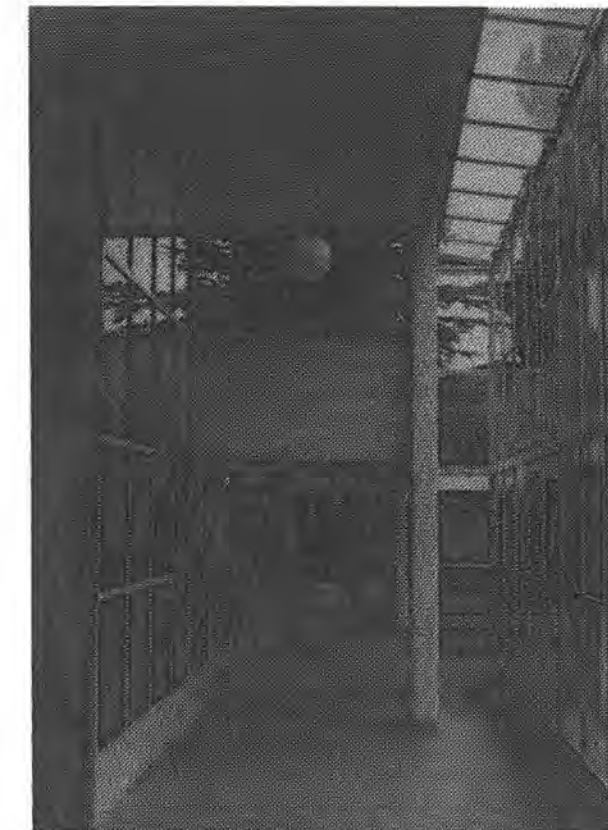
Sant' Elia School after restoration. photo by Wessel de Jonge
