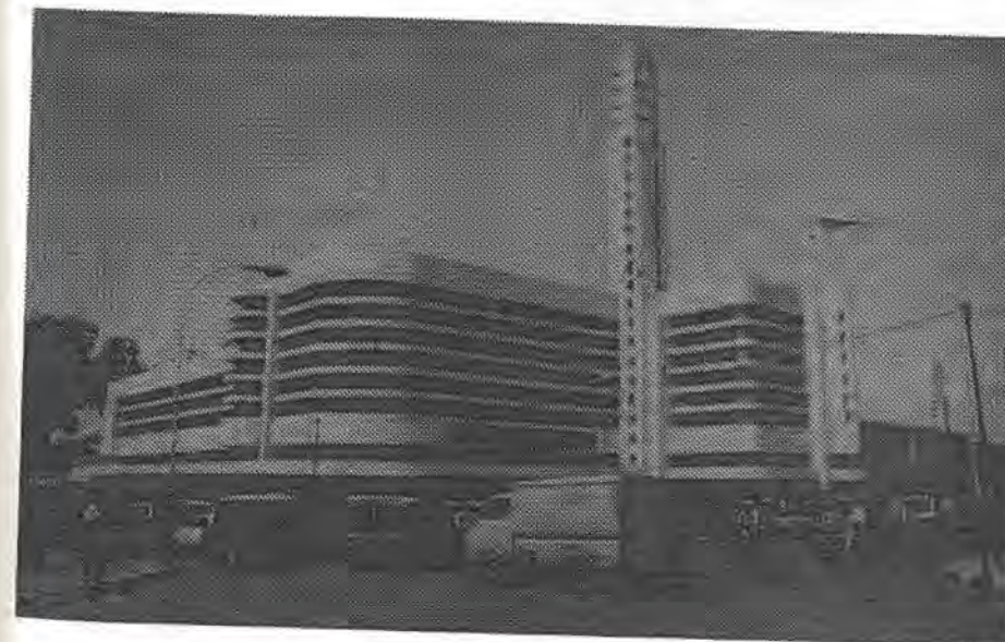
Bandung: Denis building at Jalan Braga designed by A.F. Aalbers photo: R. Gill
