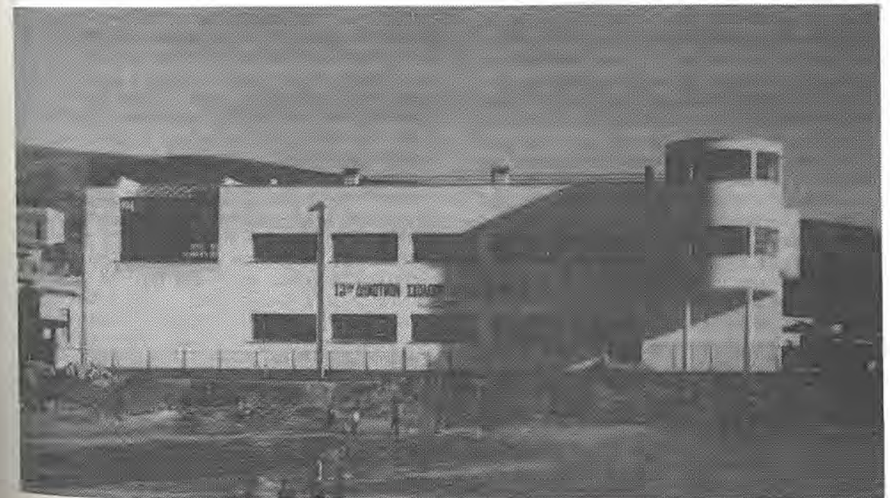
Primary School, Athens Architect K. Panayotàkos, 1933
