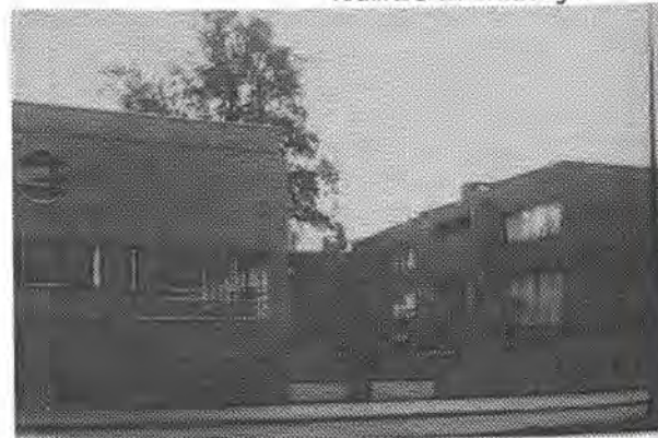
Housing complex Antwerpen Architect Van Steenbergen Archives E. van Steenbergen
