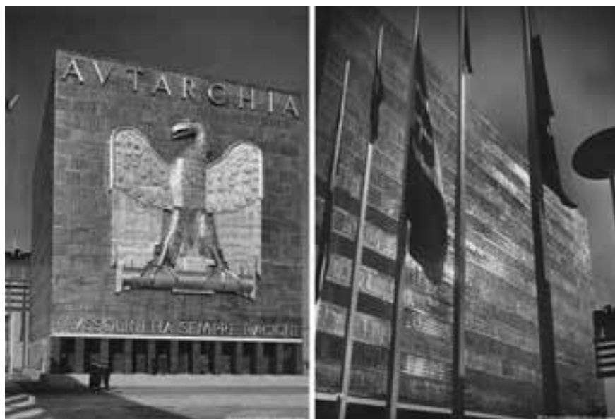
Figure 3. Autarchic Exhibition of Italian Mineral, Rome, 1938. Aluminium Pavilion, aluminium cladding façade © Montecatini Photographic Archive, Centro per la Cultura d'impresa
