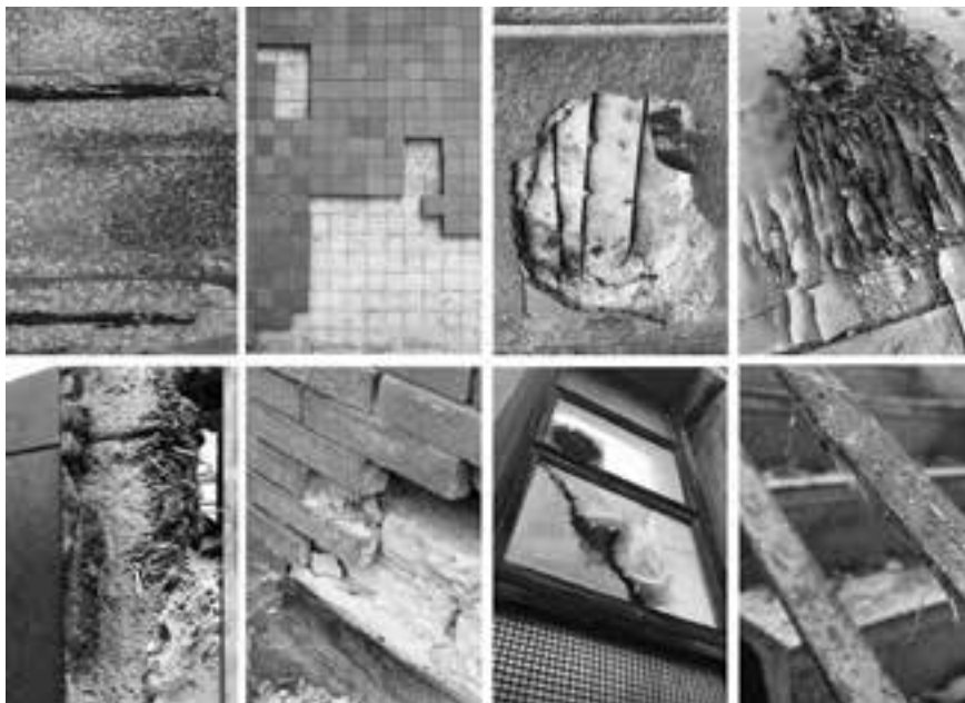
Figure 4. Autarchic materials, alteration and decay processes. From the top: artificial stone, corrosion of reinforcement and cover ejection; grès stoneware tiles, detachment and lacks; Terranova plaster, exfoliation and lacuna; Linoleum, hair cracks and burn; Eraclit panels, delamination and exfoliation; Lithoceramics, lacks and detachment of fragments; Termolux glass, exfoliation; Anticorodal, oxidation and corrosion. © Sara Di Resta 2022
