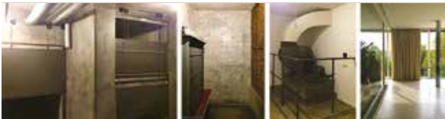
Figure 4. Ludwig Mies van der Rohe, Villa Tugendhat, Brno, Czech Republic, aeraulic system devices. © Photo: Giulia Favaretto, 2017.
