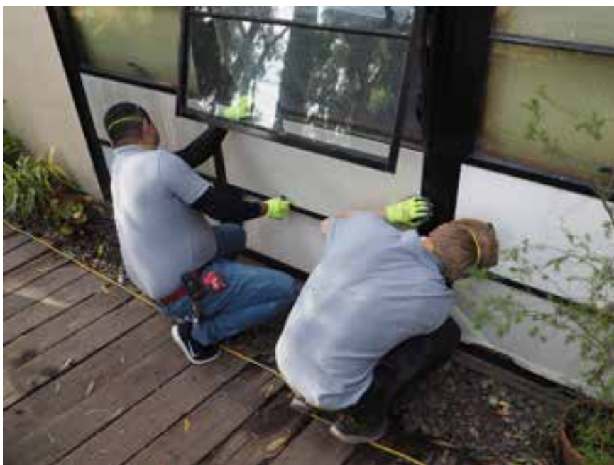
Figure 4. Architectural conservators dry-fit the panels into the steel frame and hopper window sash before final installation and sealant application, 2021. Drew Barnhart, ©J. Paul Getty Trust.
