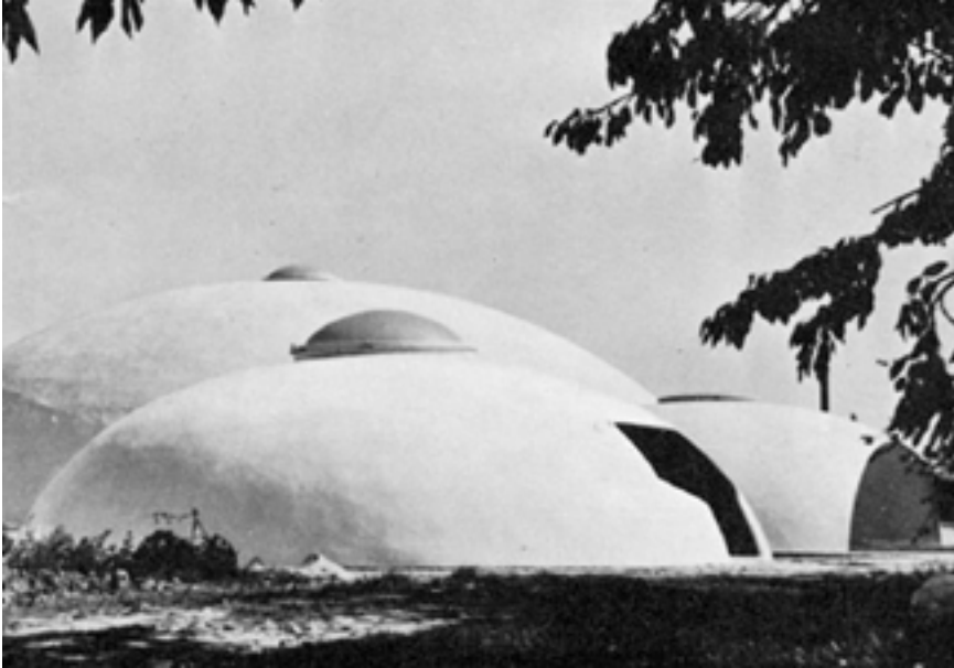
Figure 1. Dante Bini, The Mushroom field, San Cesario sul Panaro, Italy, 1965–66, The building site, domes L, I, A © Brochures from Binishells SpA
