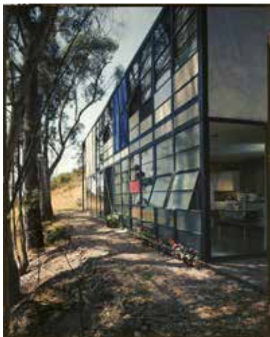
Figure 3. The Eames House, clad in a complex array of materials, including the opaque Cemesto panels, 1950. Julius Shulman, ©J. Paul Getty Trust. Getty Research Institute, Los Angeles (2004.R.10).
