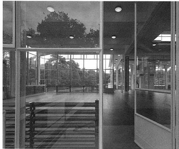
Carefully reconstructed parts such as the steel window casements, the sheet glass and the linoleum floorings. (Photo: Jannes Linders)
