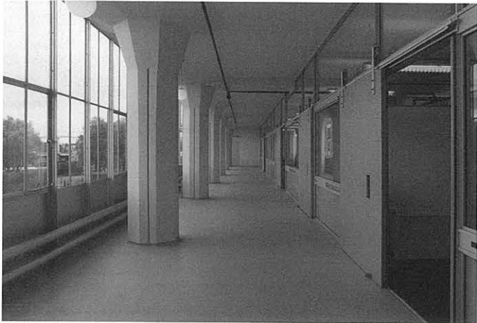
At the shadow-side, the secondary glazing is located at some distance from the original facade leaving enough space for corridors. At the other side, the sun side, the glazing has been placed between the columns, corresponding with the position of the original sunshades, creating a climate-regulating wall. (Photo: Fas Keuzenkamp)
