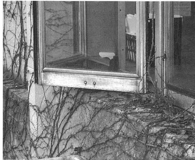
The unusual bi-fold windows at the Administration Building require frequent repairs. Parts are no longer available
