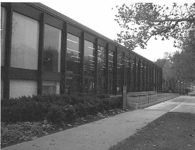
The School of Social Service Administration (Ludwig Mies van der Rohe, 1965) has experienced glass breakage from corrosion of steel elements.
