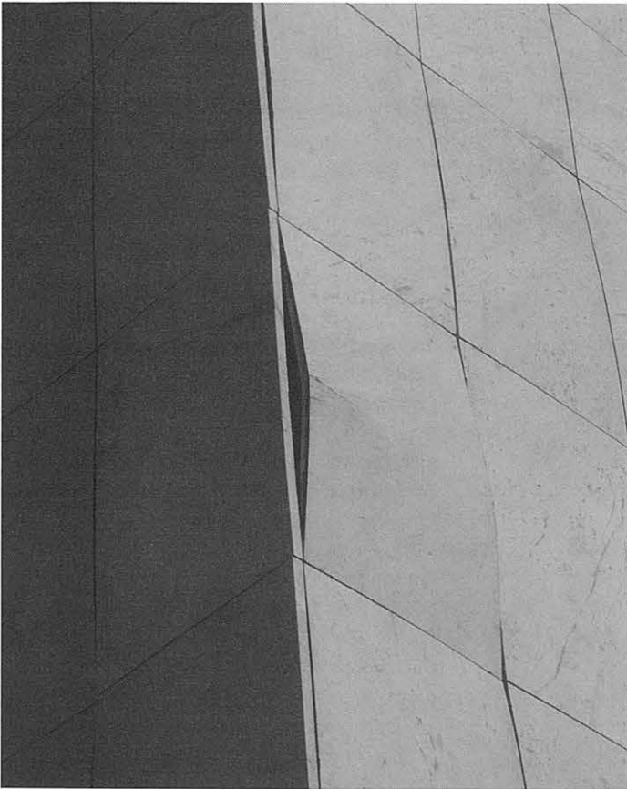
Detail of deteriorated marble on a hotel, Helsinki. (Photo: Björn Schouenborg)
