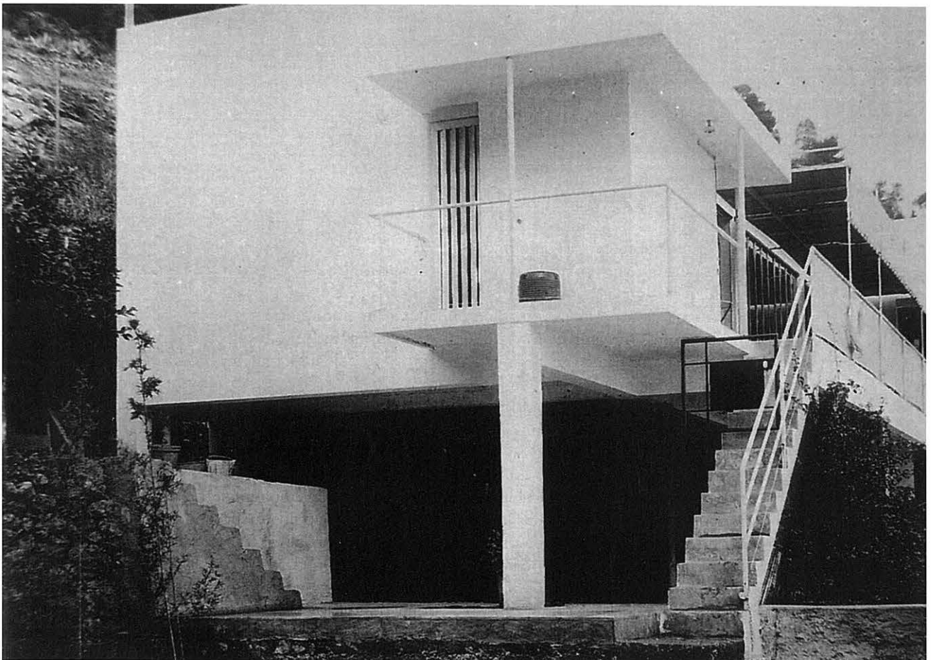
West façade. (with the small gate, seems to be strong black) From: L'Architecture vivante , 1929.
