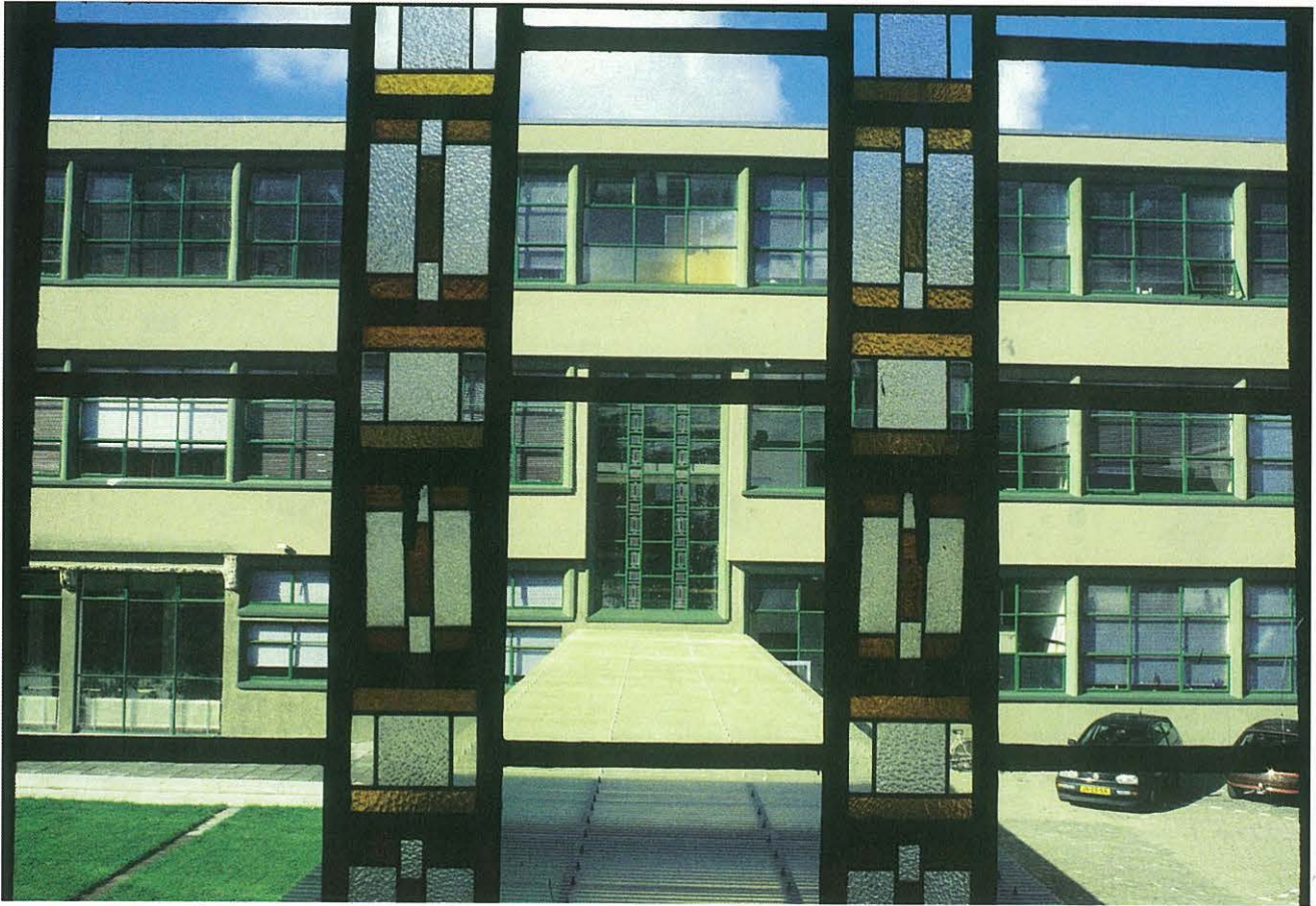
The 1922-23 Technical School in Groningen represent a threshold between traditional and modern architecture: from a decorative to a functional use of colour. Photo: W. de Jonge. ( Colour and Modern Movement architecture, by Wessel de Jonge p. 8 - p. 11 )
