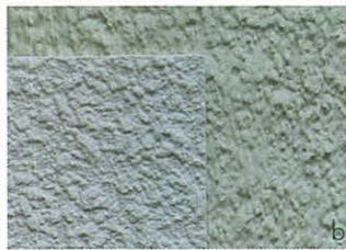
a. new standard plasterwork executed in an ordinary mechanical spray technique; right: original plasterwork (1st. phase). Photo: M. Debruyne.
