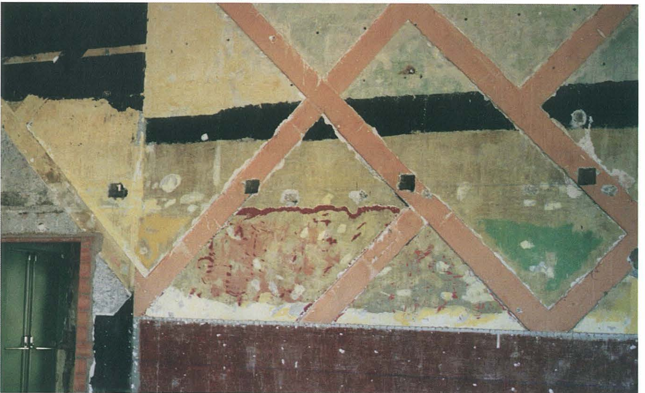
Ciné, dancing, lateral wall after dismantlement of the covering and before restoration. Photo: D. Gaymard.
