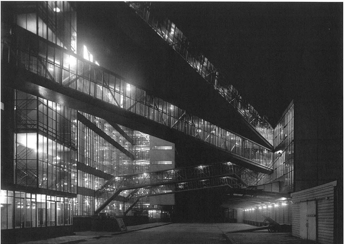
The four diagonal conveyerbridges connect the central store and dispatch department to the factories. Photo: Van Nelle Archive.
