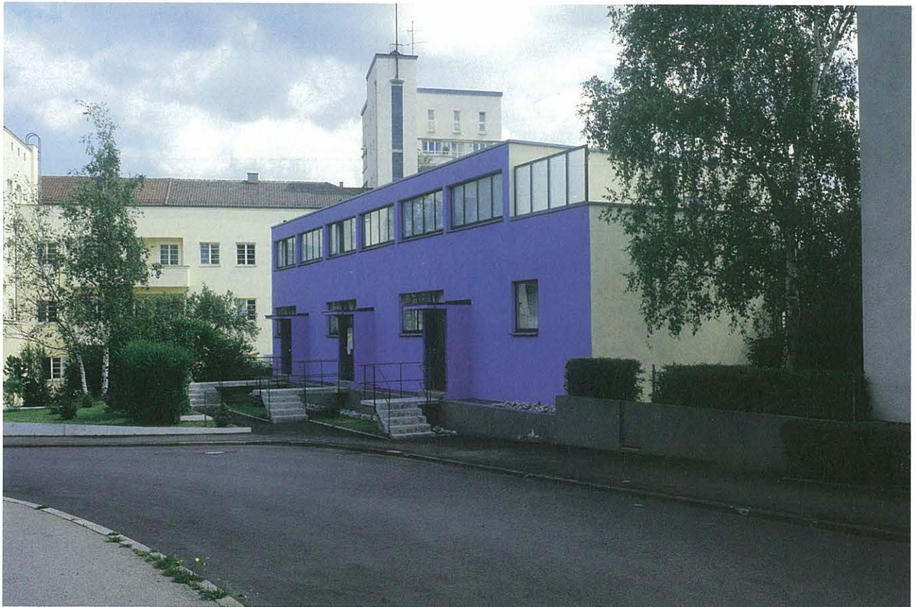
Mart Stam's 1927 terraced houses in Stuttgart reappeared after restoration with a strongly coloured north facade. Photo: W. de Jonge. ( Colour and Modern Movement architecture, by Wessel de Jonge p. 8 - p. 11 )
