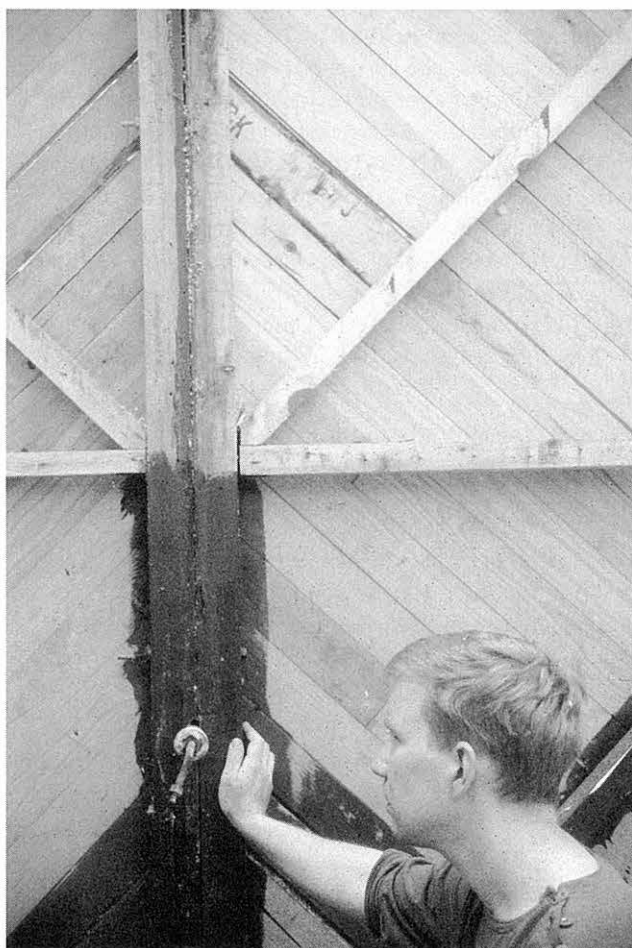
Figure 3. When the weather boarding was removed the diagonal bracing and the cross-wise inner boarding became visible.
