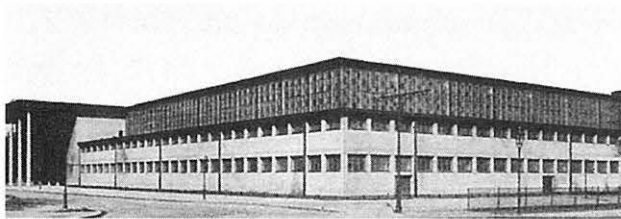
Fig. 1-3. Messehof in Breslau, 1924. Design by Max Berg. Solid-web girders construction manufactured by the firm Tuchscherer Inc.. Parabolic two-hinged arches with a span of 37.60 m.
