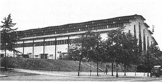
Fig. 18 to 20. Sport arena in Stuttgart/ Germany, 1925-1926. Design by Hugo Keuerleber. Framework by the firm Karl Kübler Inc. from Stuttgart/ Germany. Three-hinged frames with a span of 50.00 m.
