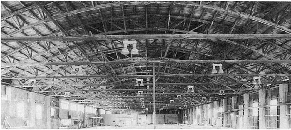
Fig. 10. Planer-hall in Magdeburg/ Germany; built by the firm Karl Kübler Inc. from Stuttgart in 1923. Two-hinged frames with a tie-member with a span of 33.40 m.
