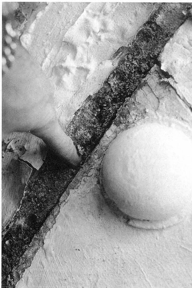
Figure 2. The timber of the triangles was in many parts totally decomposed by funghi, thanks to the hard thick plastic paint.
