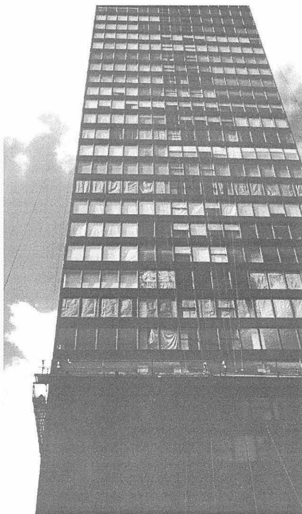
Full scale curtain wall removal and recladding has become a popular repair choice. In this case, curtain wall removal and replacement is occurring simultaneously.
