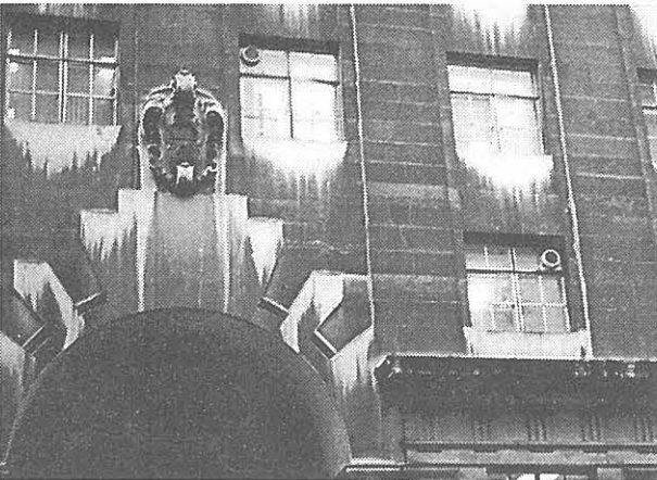
Reuters Building in Fleet Street, London. The typical streaking effect seen in Portland Stone, is due to general dirt discolouration and localised washing, where water runs down face of stone.
