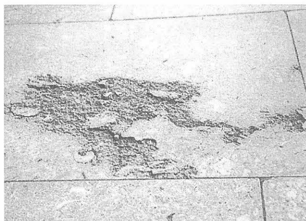
Spalling damage due to weathering to facebedded Derbyshire.
