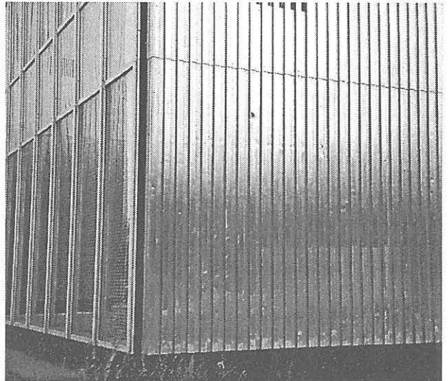
The dented Remanit panels on the end facade are witnesses of the past and add a pleasant flavour to the renovated Thyssen Haus. Photo: Wessel de Jonge (1996).
