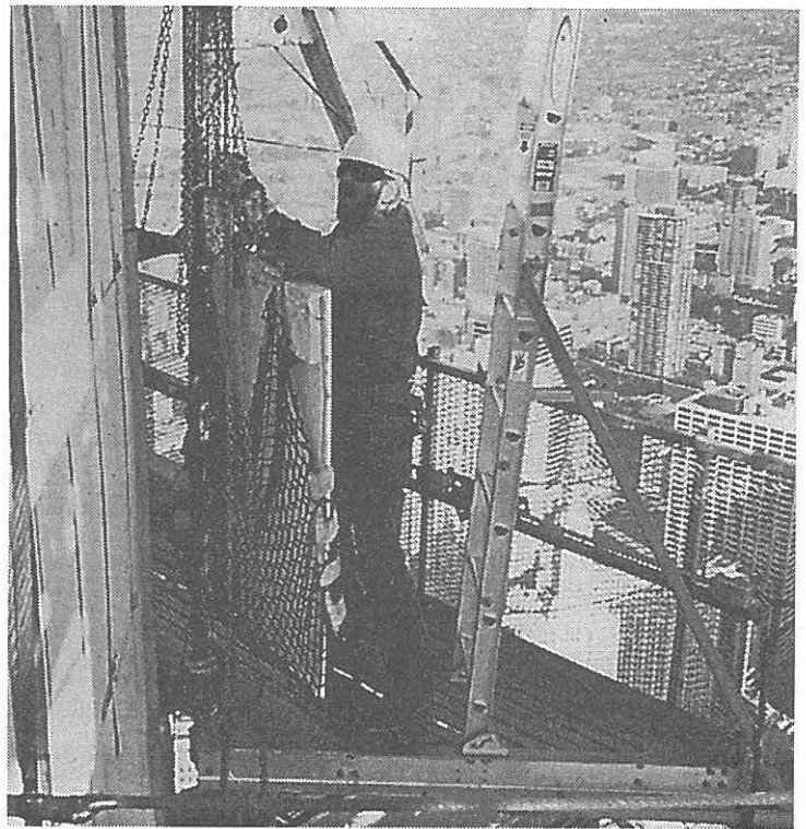
Marble panels being removed from the Amoco facade high above the streets of Chicago's Loop. Photo: Wiss, Janney, Elstner Associates, Inc.
