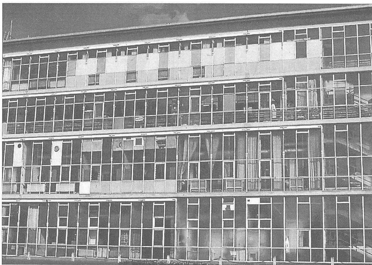
The Boots Factory with original glazing before renovation, with opening lights and structural mullions between the three window bays.
