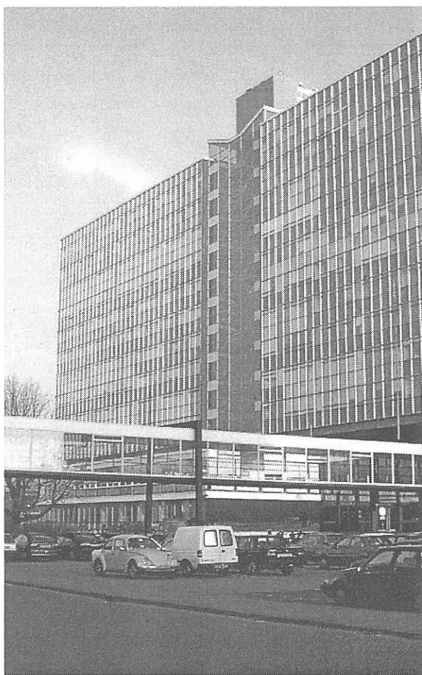
The main building of the Eindhoven University of Technology features a typical early postwar curtain wall. The staircase has been recently refurbished and displays a much more smooth facade. Photo: Patrick van Buijtenen.
